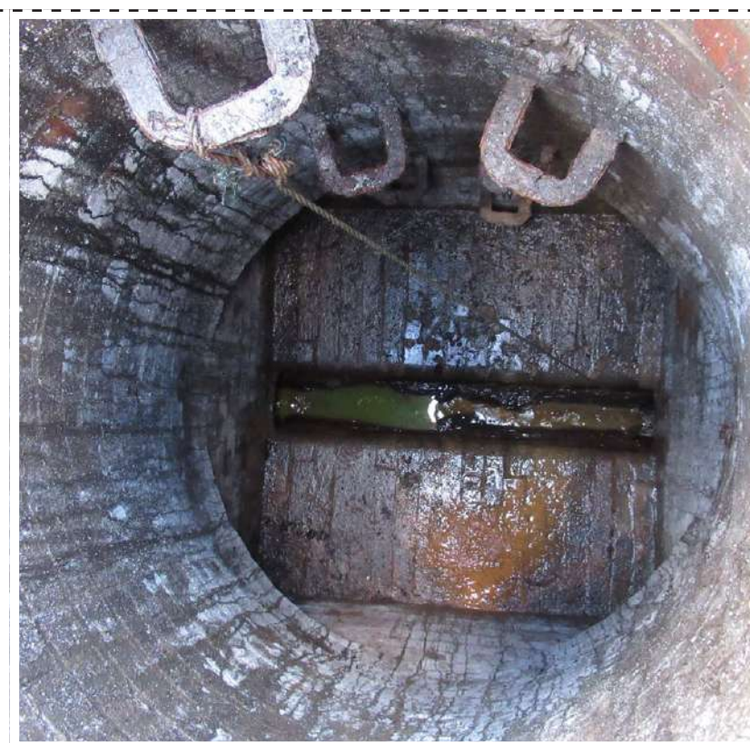
Fig. 16: Tracer dye from the field corner chamber appeared in the road system.
