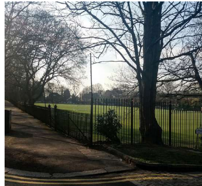
Fig. 7: Disused pedestrian access gate off Hampstead Lane
