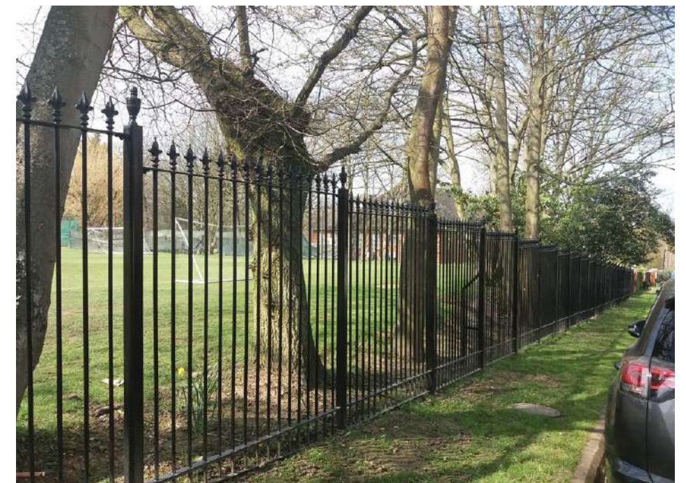
Fig. 12: New fencing installed in 2019 along Courtenay Avenue
