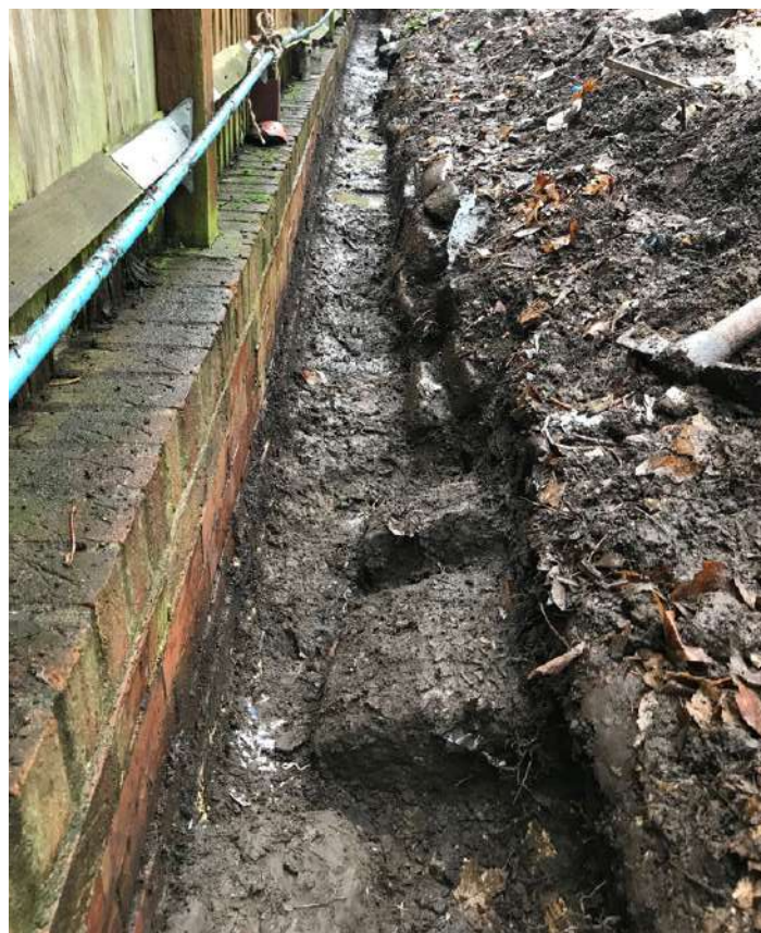
Fig. 13: The remains of the stone-block lined ditch, later brick wall and concrete bed.
