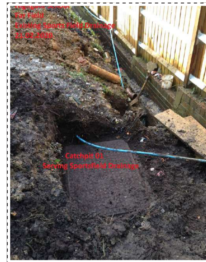
Fig. 15: The exposed outfall chamber cover with inflow land drainage pipes & outflow to the road system.
