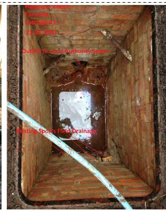
Fig. 15: The exposed outfall chamber cover with inflow land drainage pipes & outflow to the road system.
