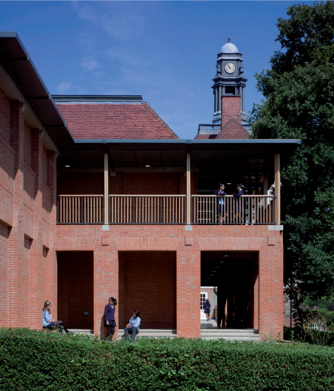
The Henrietta Barnett School, London, Hopkins Architects
