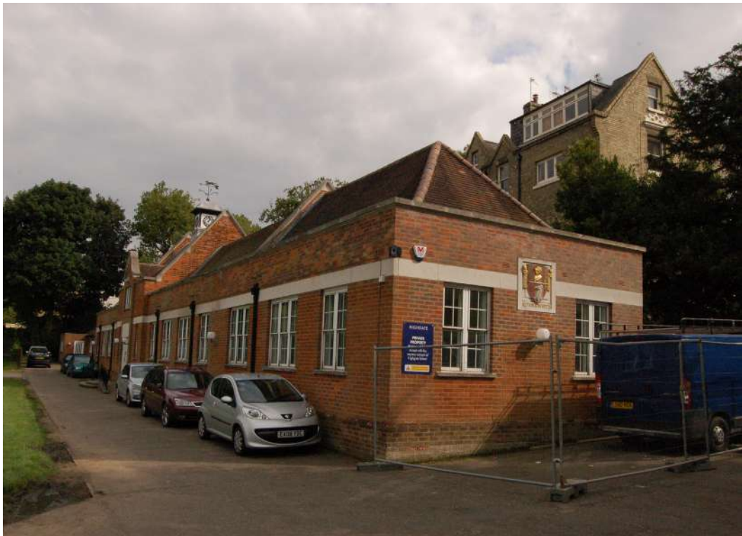
2. Existing car parking to west
