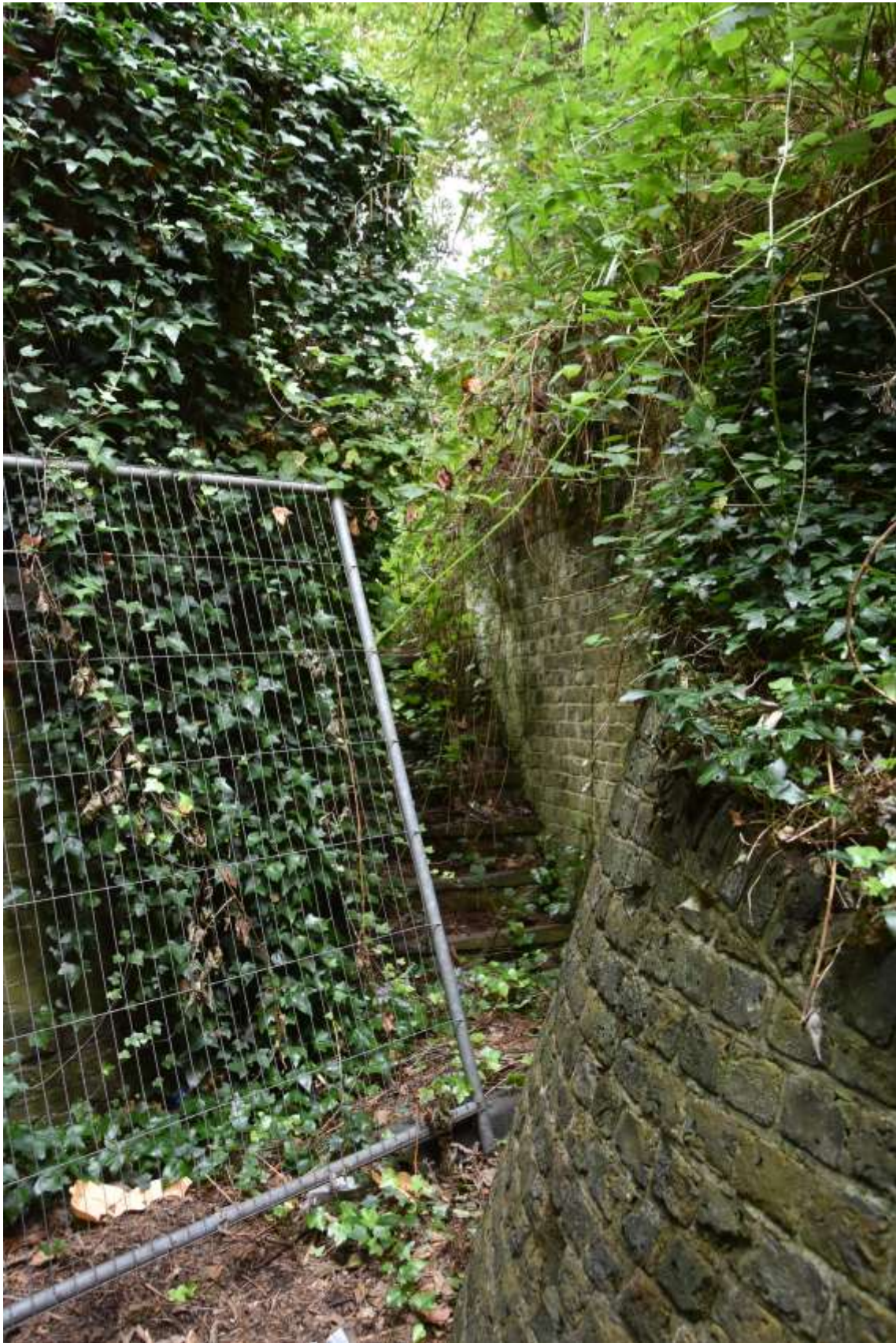
Fig.41: Steps and retaining wall on the north side of Parade Ground Building, facing SW
