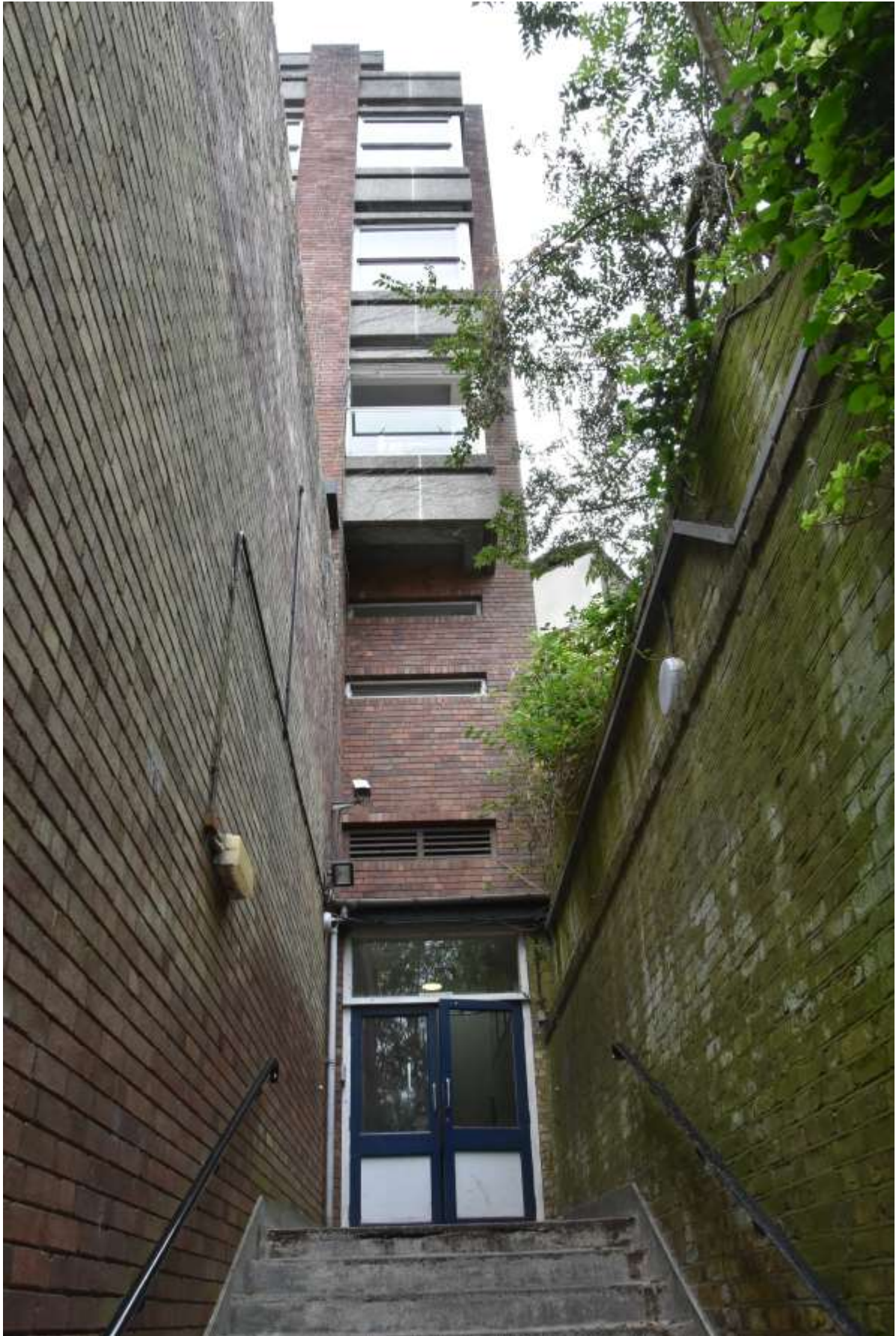
Fig.29: Rear exit of Dyne House to The Gibbon Garden level. The roof terrace lies two floors up from the bottom of the steps, to the left of frame. Facing SW
