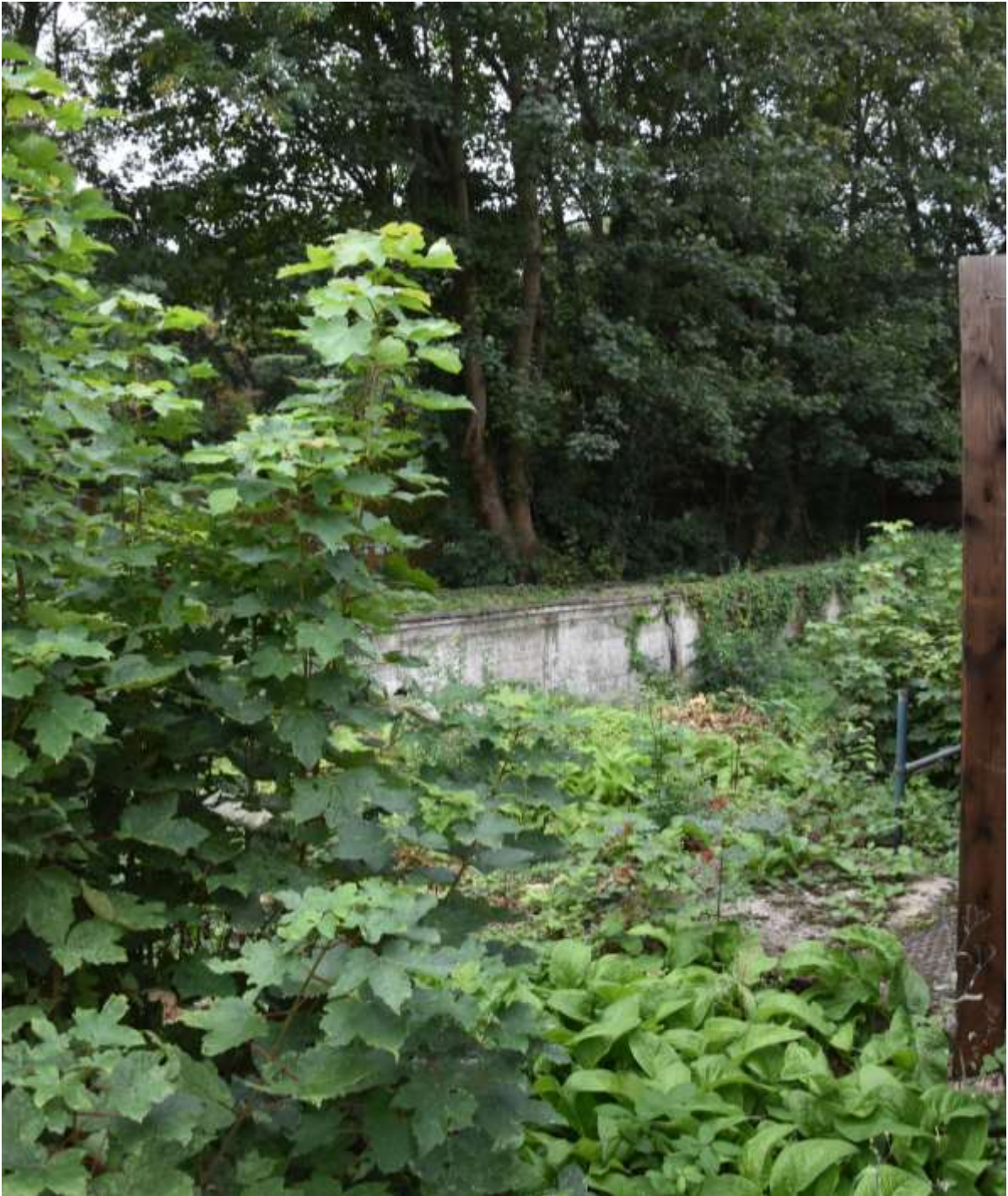
Fig.38: Redundant 1950s swimming pool facing S
