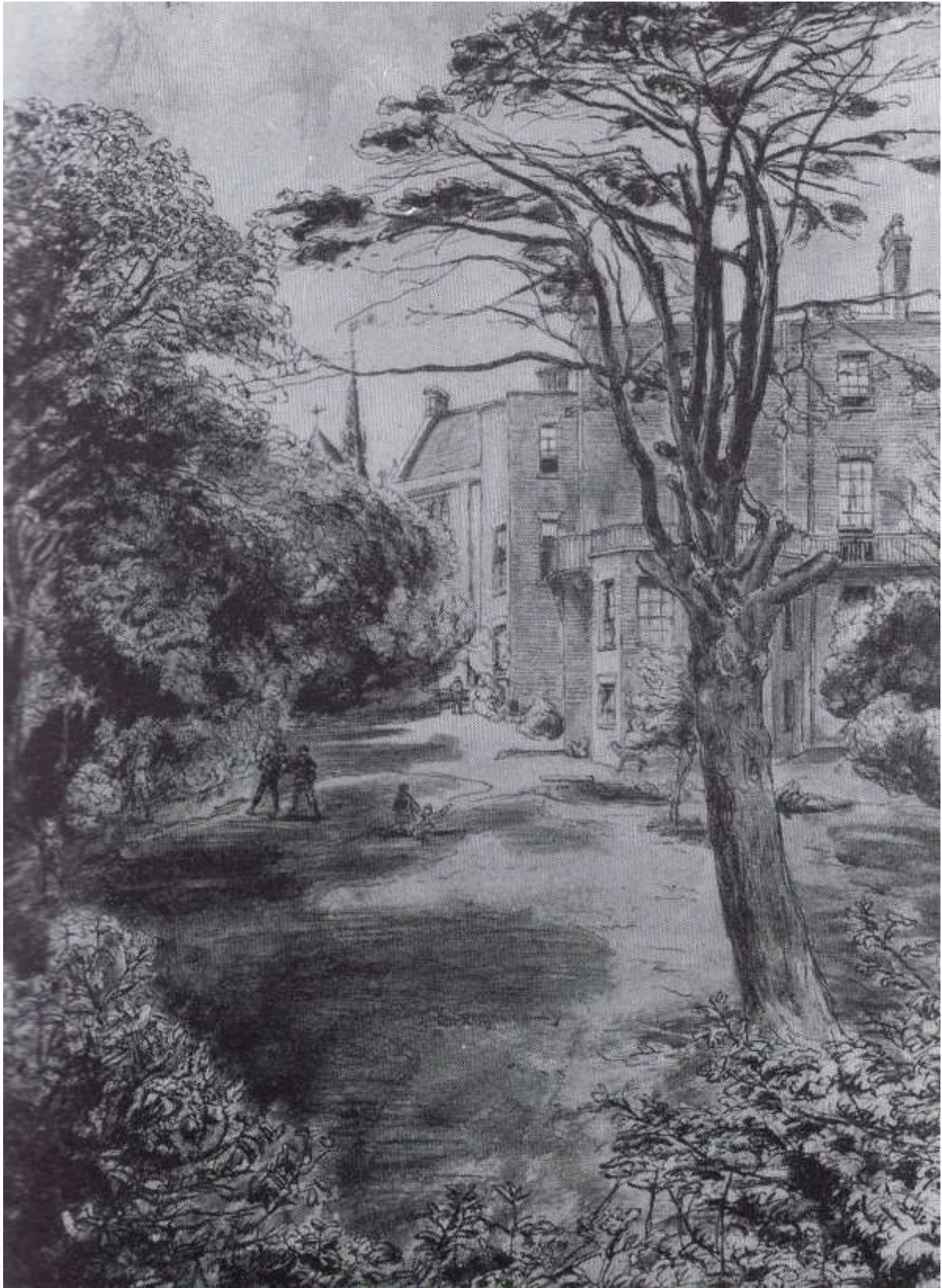
Fig.20: Rear view of the Old Dyne House facing SW, before its demolition in 1966. Highgate Chapel is just visible above the tree-line in the background
