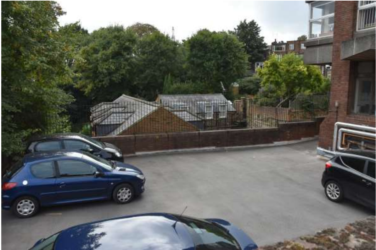
Fig.28: Roof terrace car park, facing S. Note the adjoining properties built downslope, denoting the significant drop-off
