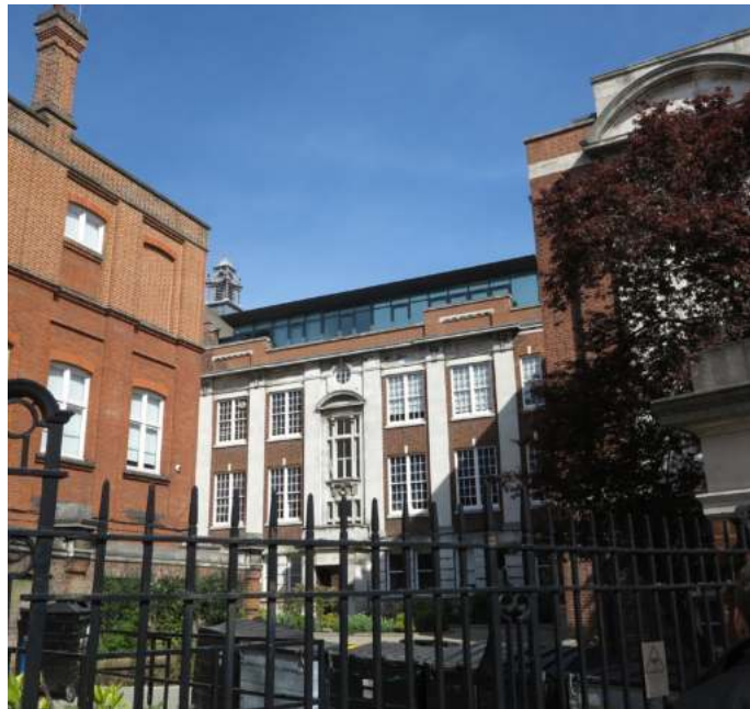
2. The Science Building 1928
