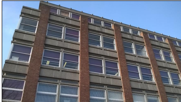
Photo 6: The eastern elevation of B2.
