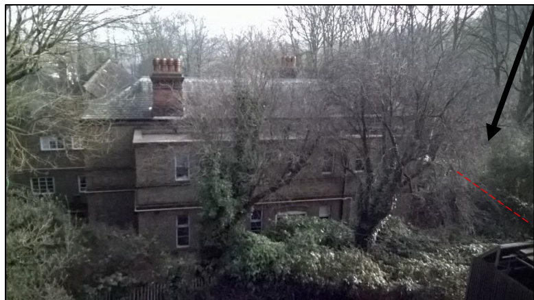
Photo 3: The eastern elevation of B1 (arrow)
