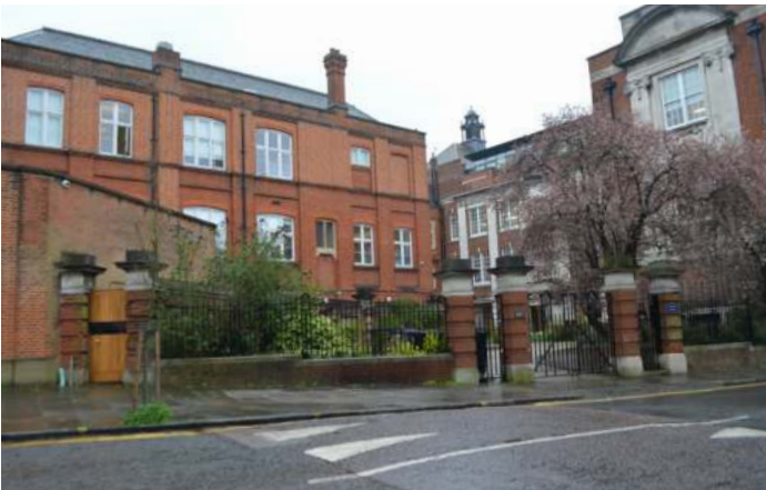
1. View from Dyne House across to the Science Quad
