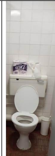
Image 14 Washroom Tiles and WC's
