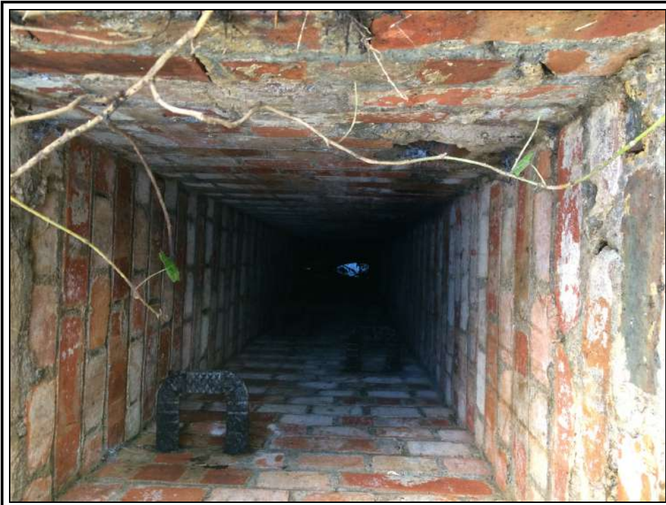
Photo 6, View down MH04
