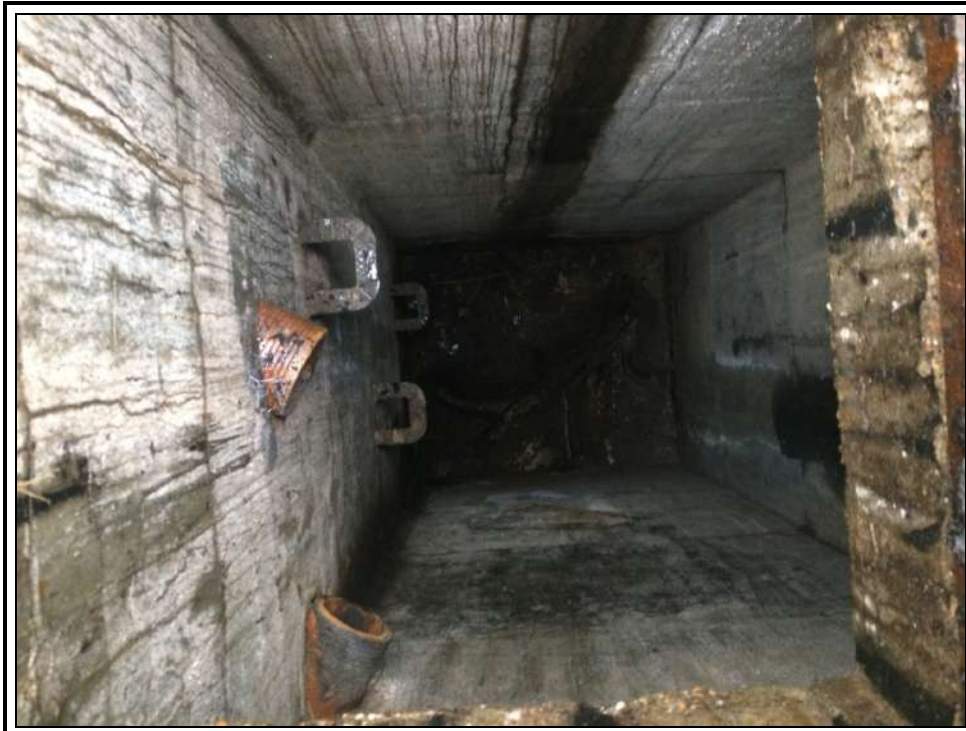
Photo 8, View down MH05
