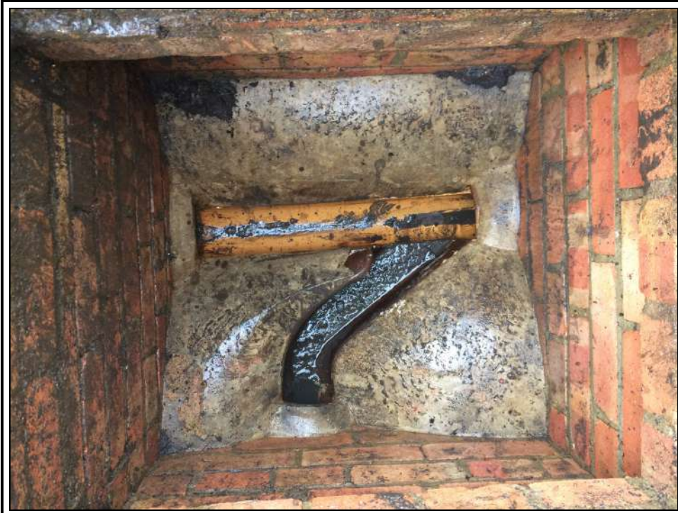
Photo 15, View down MH10
