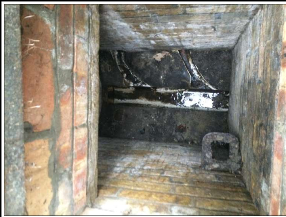
Photo 4, View down MH03
