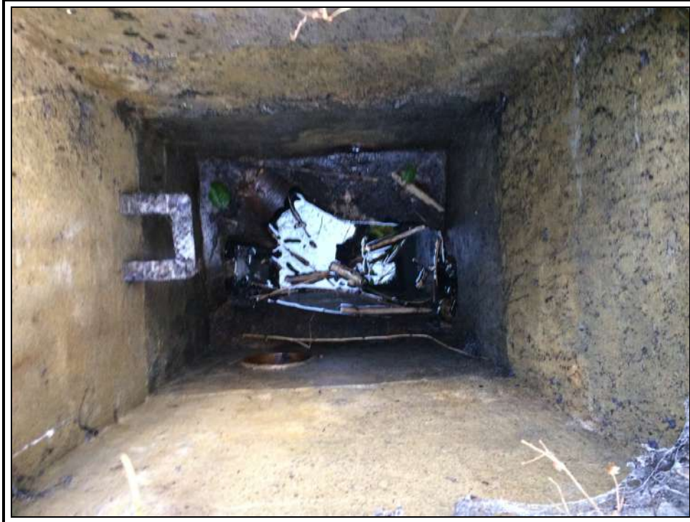
Photo 11, View down MH07
