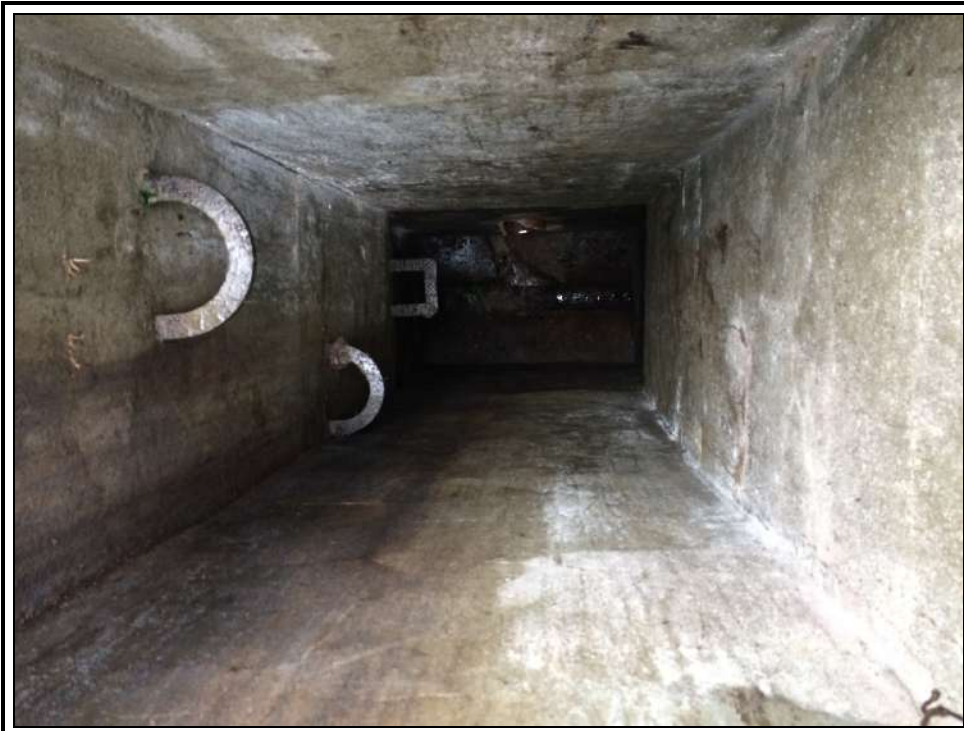
Photo 10, View down MH06
