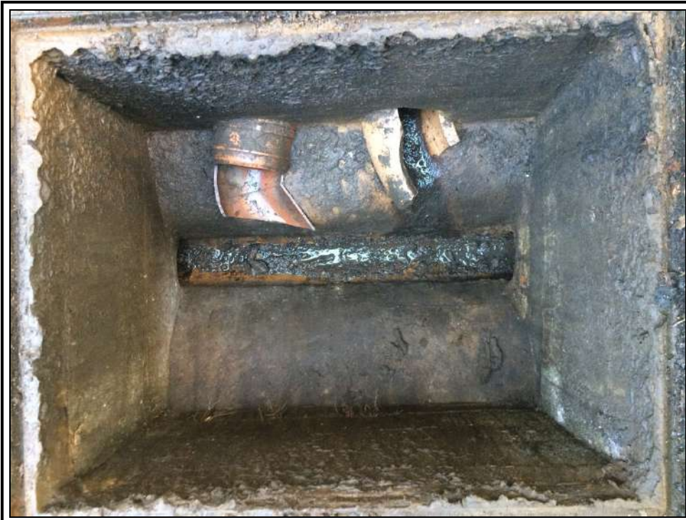
Photo 2, View down MH01
