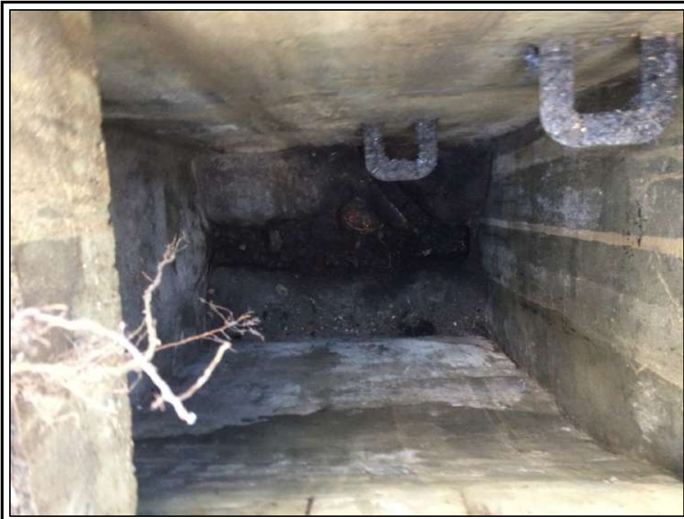
Photo 13, View down MH08
