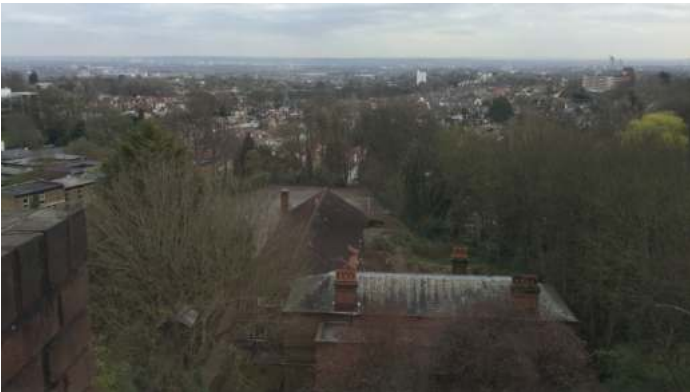
View from Dyne House looking towards the Parade Ground
