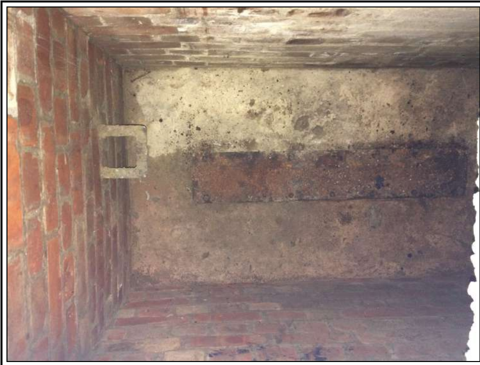
Photo 17, View down MH11
