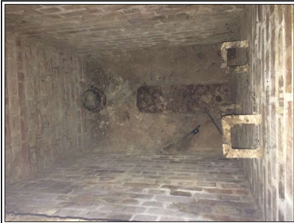
Photo 23, View down MH14
