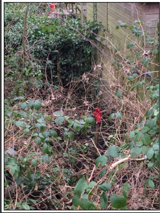
Photo 32, Location of downstream chamber or Main of MH07
