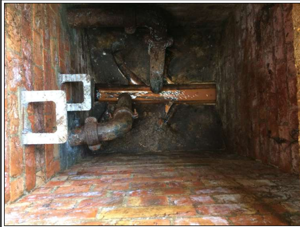
Photo 27, View down MH16
