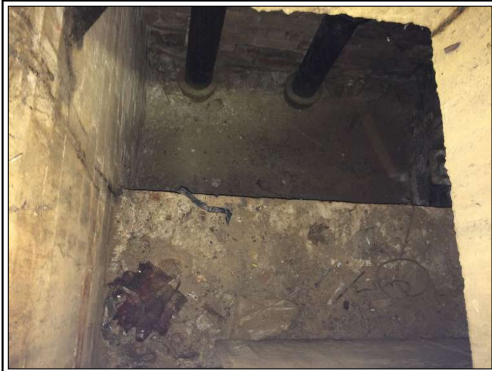
Photo 21, View down MH13
