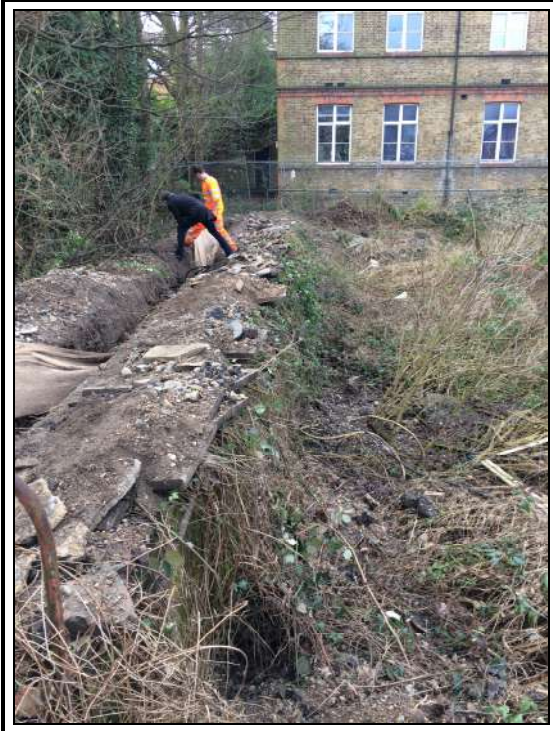
Photo 36, General site photo
