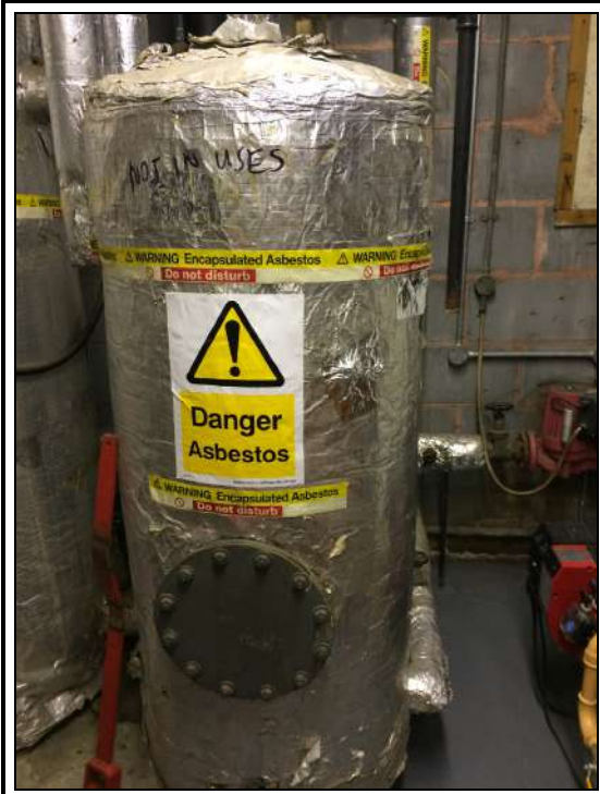
Photo 33, General site photo
