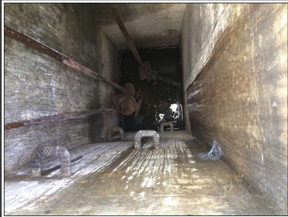
Photo 31, View down Valve Chamber
