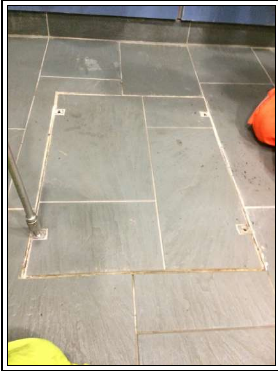
Photo 18, Location of MH12 - UTR
