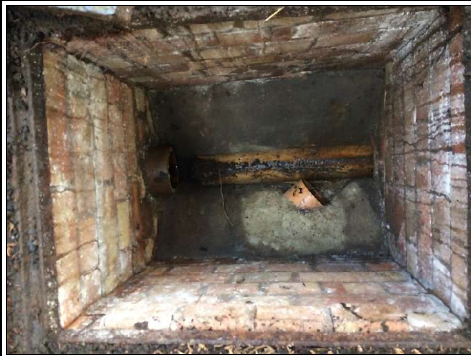
Photo 29, View down MH17
