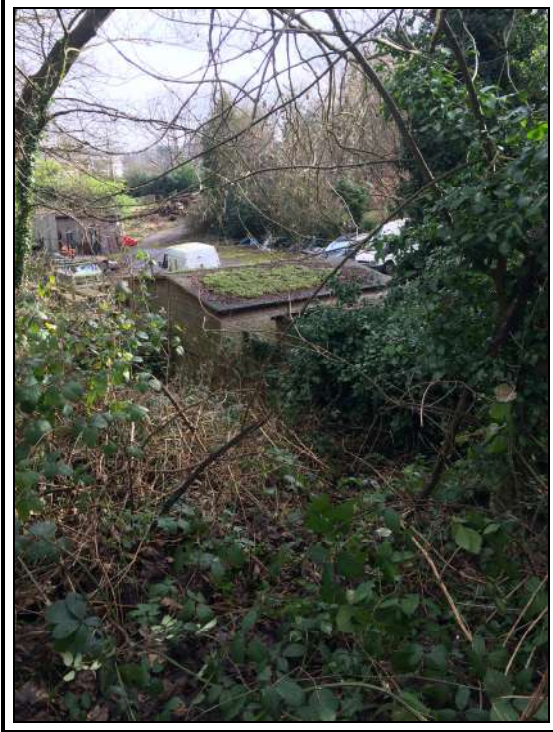
Photo 34, General site photo
