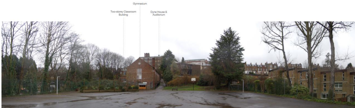
Figure 3 Class Room Building, Gymnasium and Dyne House and Auditorium
