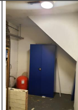
Image 19 Classroom Building, Gymnasium and Swimming Pool - Plasterboard
