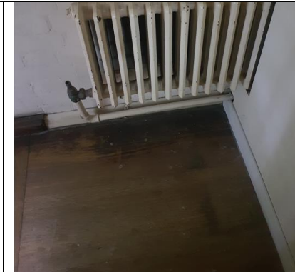
Image 13 Classroom Building, Gymnasium and Swimming Pool - Fibre Board
