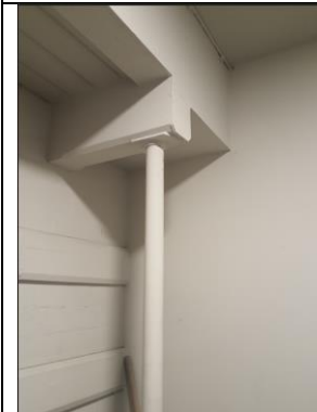
Image 20 Island Site Tunnel - Plasterboard
