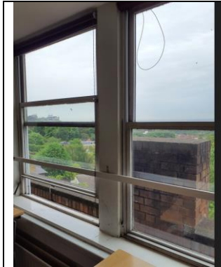
Image 10 Dyne House - Aluminium Window Frame
