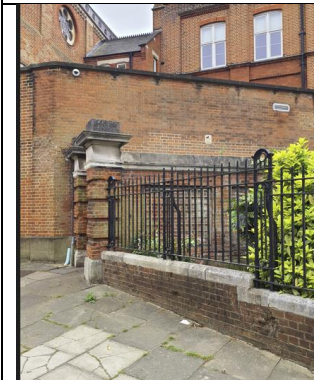
Image 7 Island Site Tunnel - Brick Wall (External)
