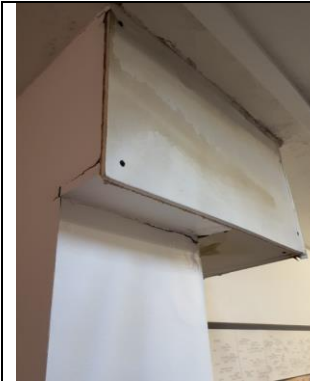
Image 18 Dyne House - Plasterboard
