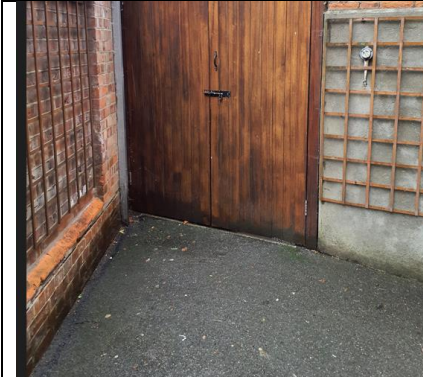
Image 29 Island Site Tunnel - Hardstanding
