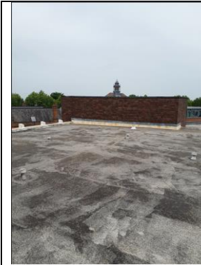
Image 27 Dyne House - Asphalt Roof
