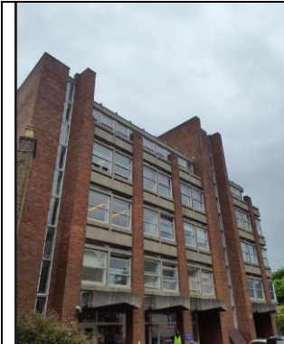
Image 5 Dyne House - Brick Wall
