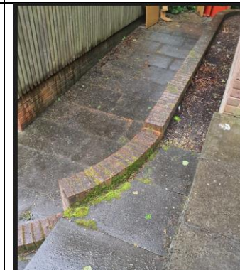
Image 8 Gibson Garden - Bricks Wall (External)
