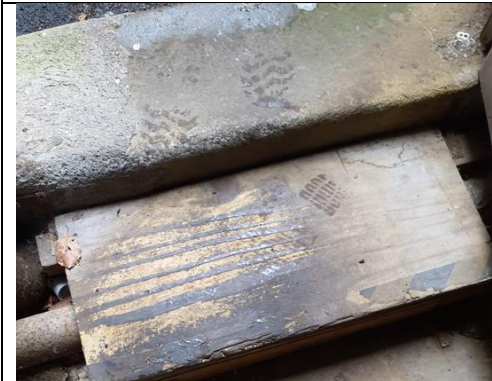
Image 3 Island Site Tunnel – Concrete Slab
