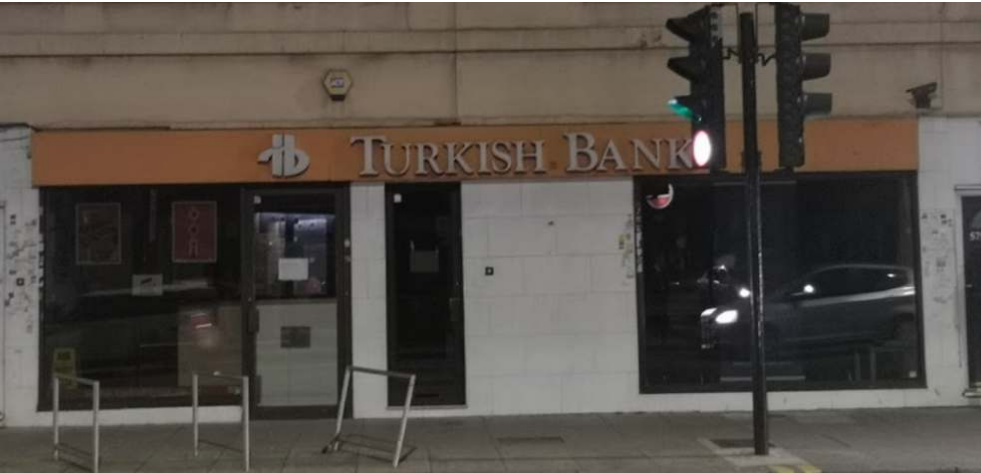
Existing Signage - Approx Height from ground 2.4m Size - 9015mm x 530mm
