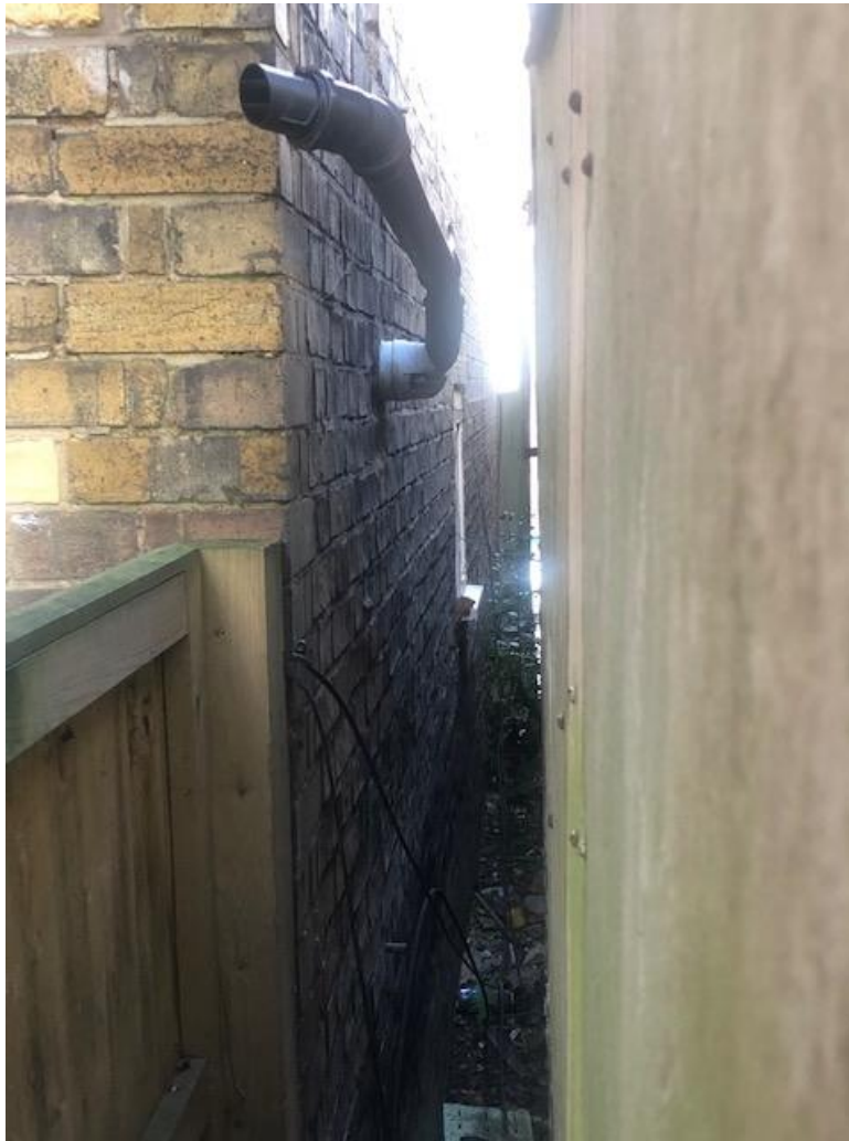
Photo of window down side elevation
