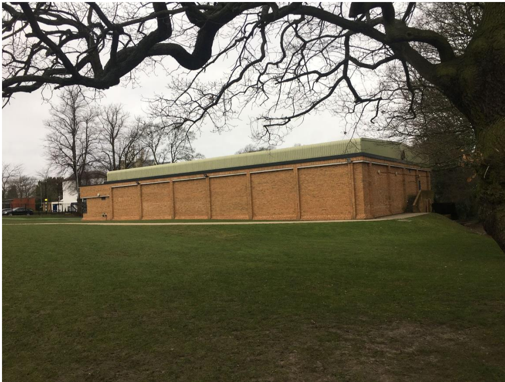
Figure 26. View of side and return elevation of the Mallinson Sport Centre. Note blind brick façade contributing a plain utilitarian appearance to long range views across the playing field.
