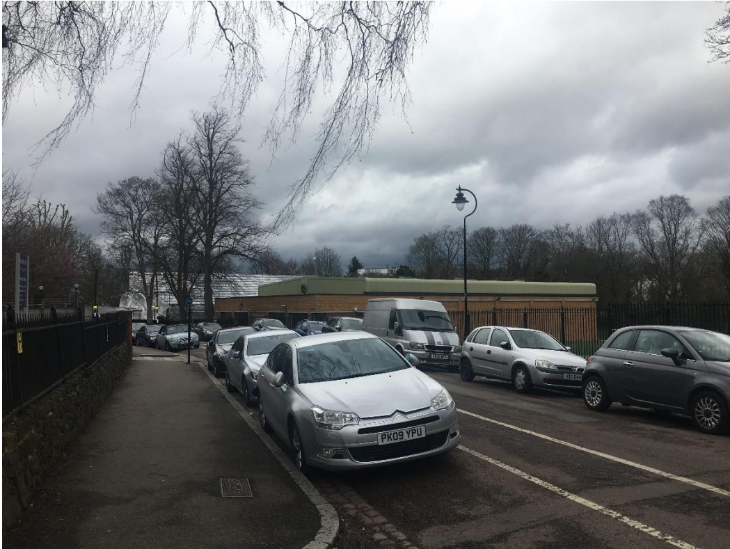
Figure 32. View of Mallinson Sport Centre from the south, with swimming pool seen to the rear, currently undergoing refurbishment works.
