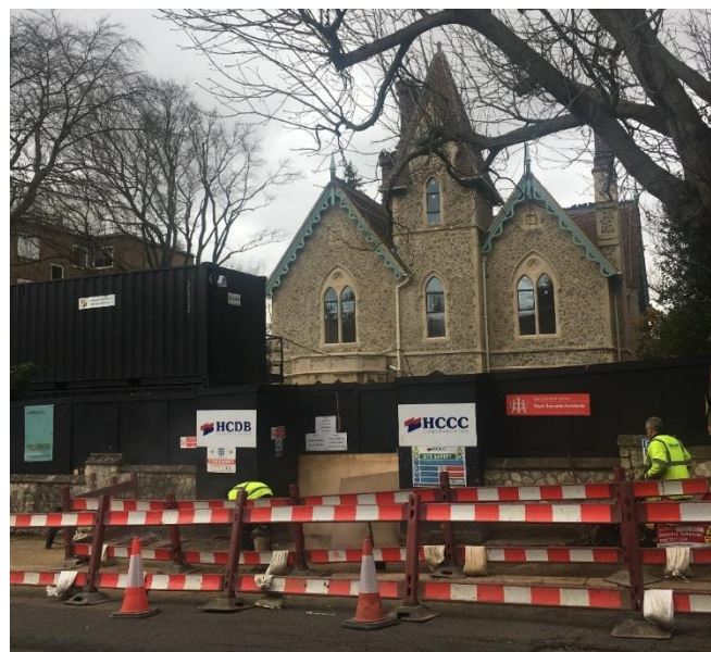
Figure 35. View of 16 Broadlands from Broadlands Road. Note works partially covered views of the building at time of site visit.
