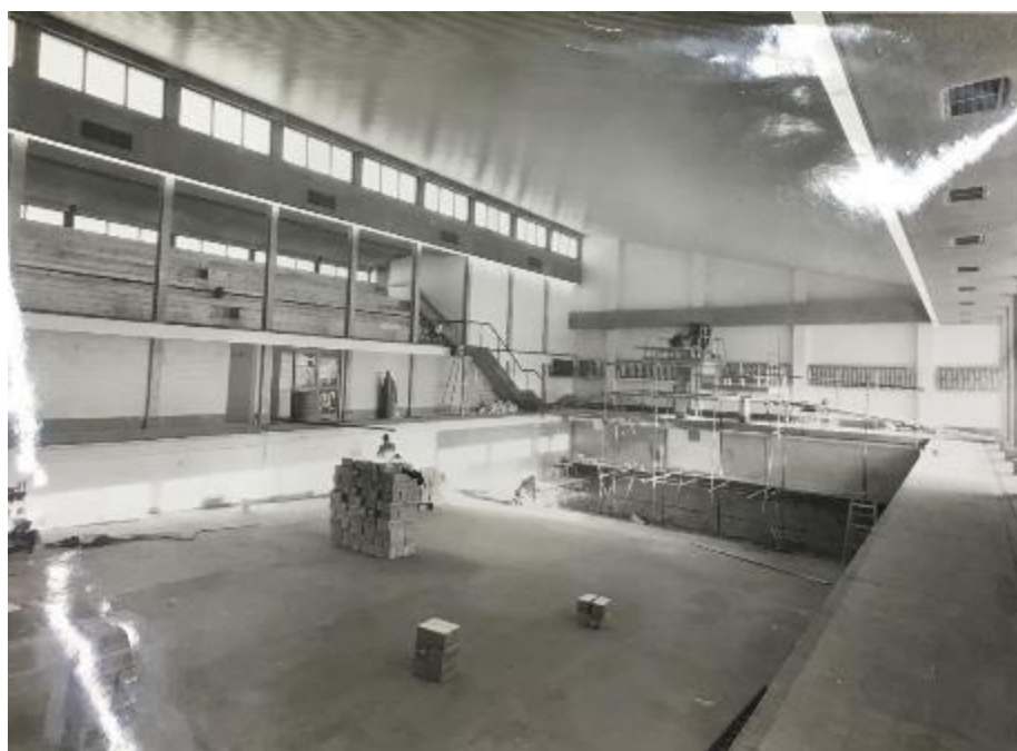
Figure 14. Mallinson Swimming Pool Under Construction.
