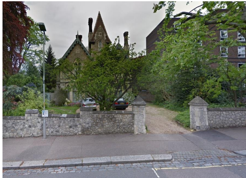
Figure 38. Grade II listed forecourt wall to 16 Broadlands Road.
