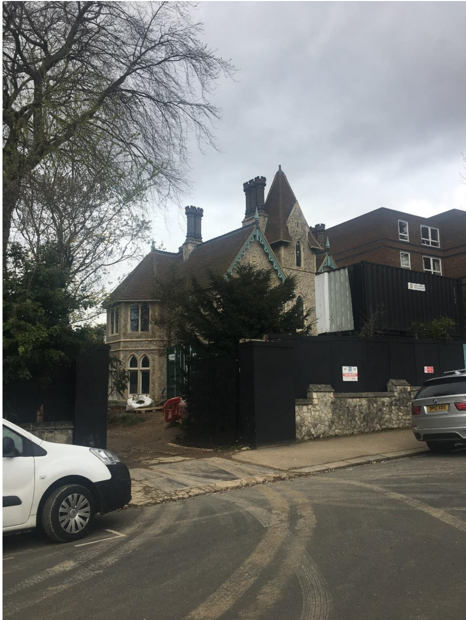
Figure 36. View of 16 Broadlands Road seen from the road.
