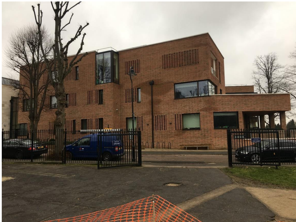
Figure 29. Contemporary extension in the location of the now demolished Cholmeley House. Note use of decorative brick ventilation panels as well as asymmetric fenestration pattern.
