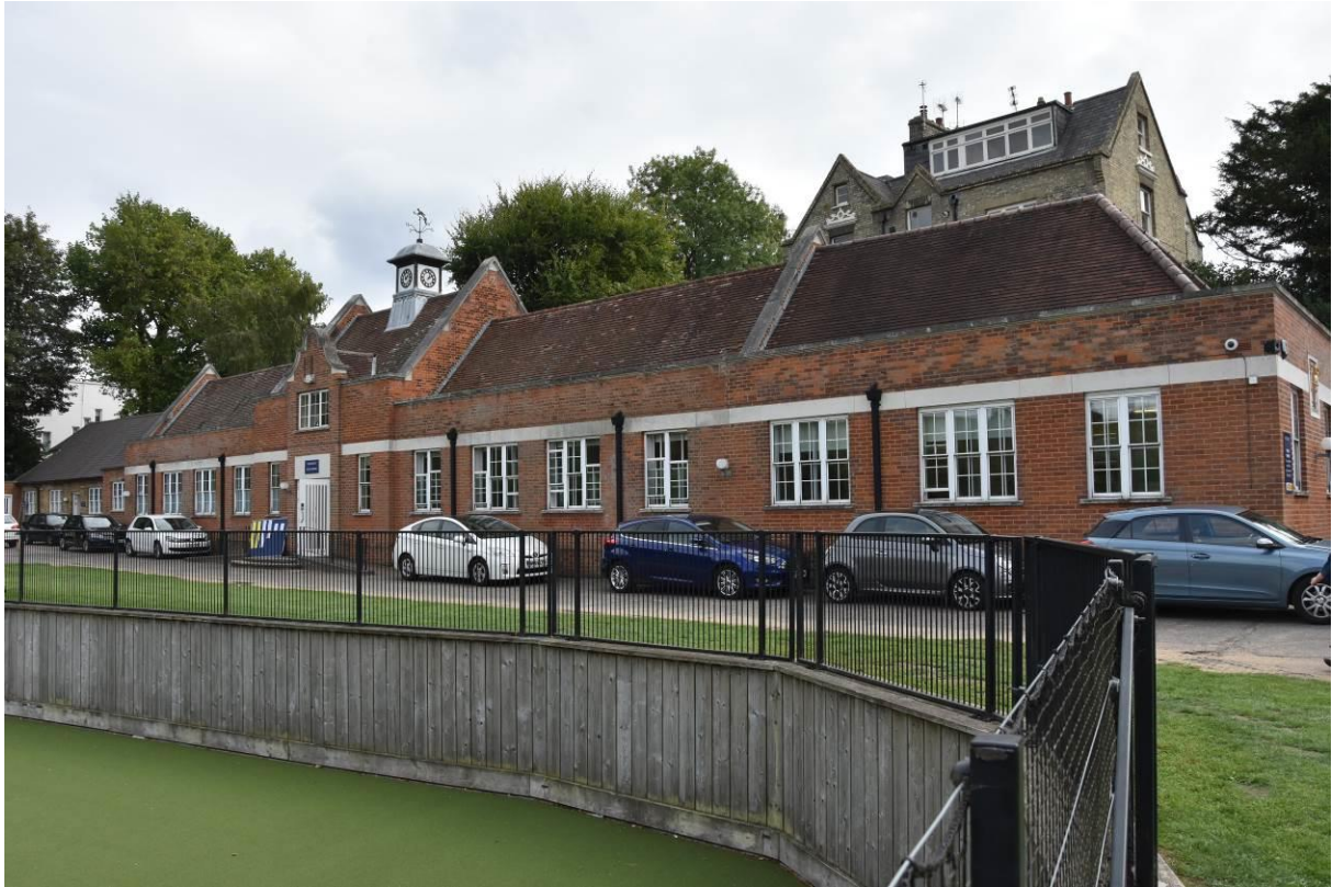
Fig.27: Terraced ground of all-weather pitches and southern retaining wall, facing SE
