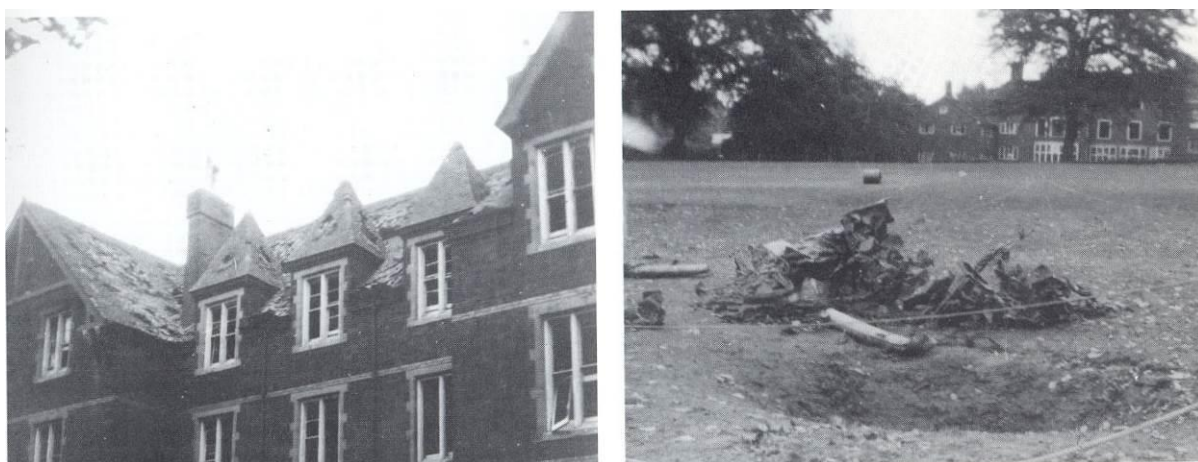
Fig.19: Photograph of the V1 Crater (right image) and damage done to the School House (left image) – reproduced from Hinde, 'Highgate School'
