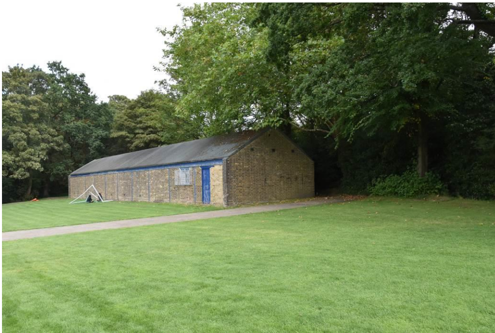
Fig.31: Rifle-range building in the northeast corner of the Junior playing field, facing NE
