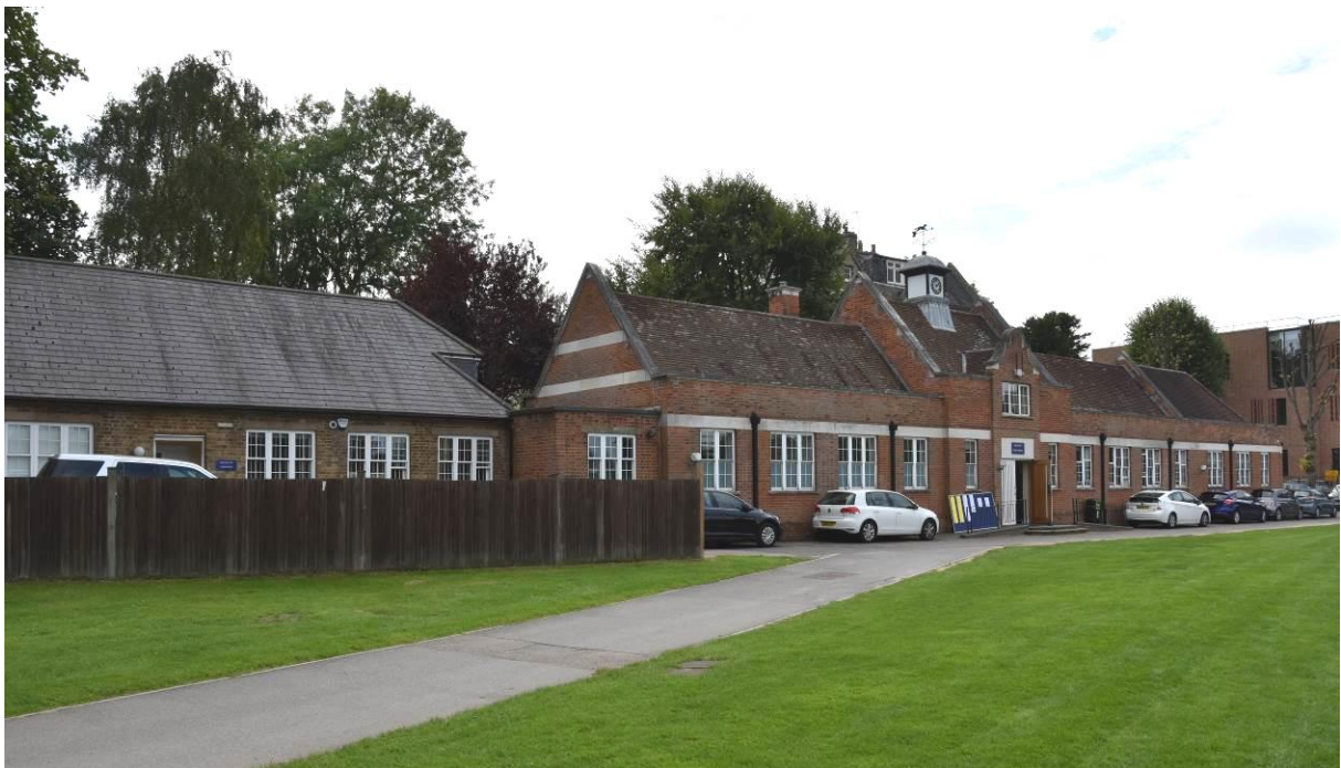
Fig.25: Richards Music Centre, facing WSW. Note that it is converted from the two separate buildings which were labelled Pavilions in the 1930s
