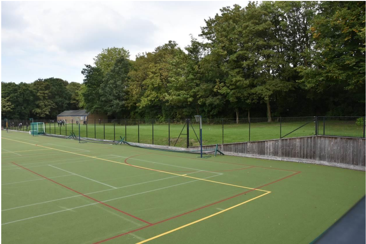
Fig.26: The all-weather pitches terraced into the natural slope, note the retaining wall to the west, (top of frame), facing NE
