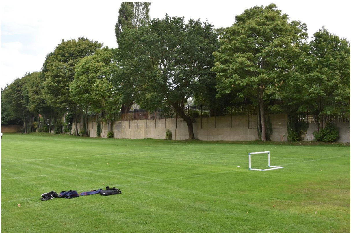
Fig.36: West side of 'Tatham's Field' showing the eastern retaining wall, facing NE
