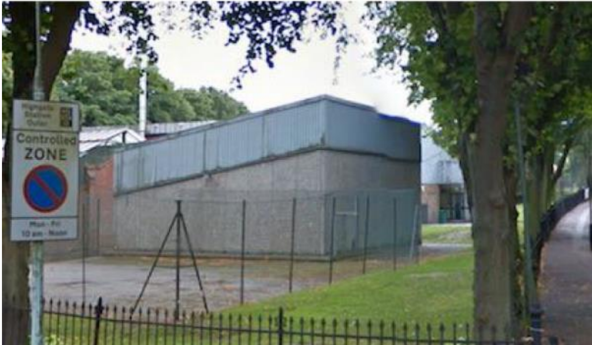
Figure 3 Northern Squash Courts
