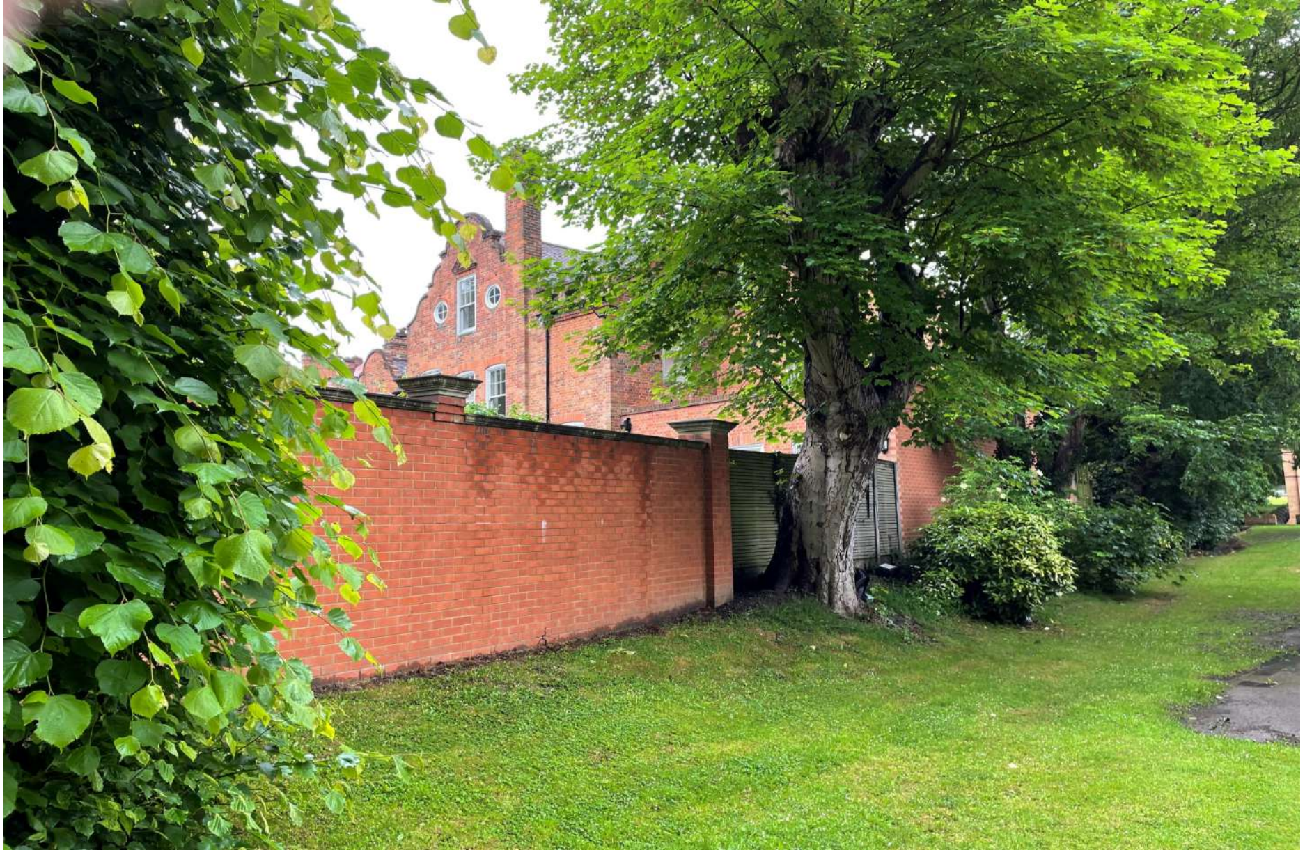
Photo F - Boundary Wall to No 27 Broadlands Road
