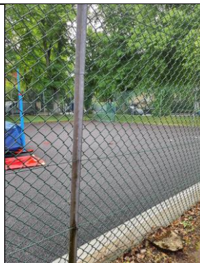
Image 7 Mixed Metal Fence
