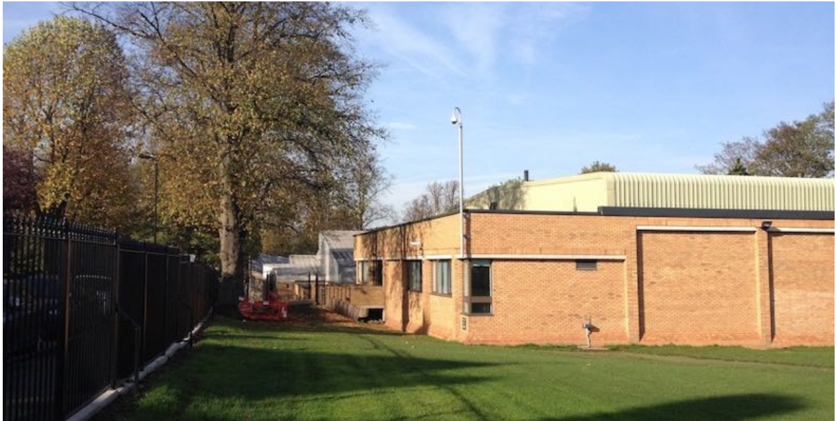
View of the MSC sports centre site from south
