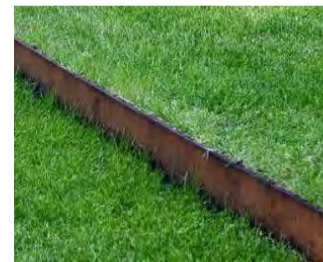
STEPS&SEATS - SPORTS PITCH FLOOD BASIN Corten steel edge restraint for sports pitch flood basin seats and steps
