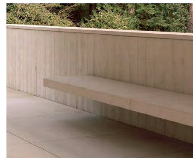
SEATS - FIVES COURTS Cantilever concrete seat
