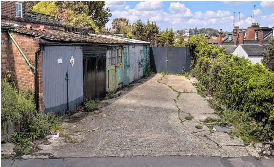
4. VIEW OF 60 WOLSELEY ROAD FLANK WALL & GARAGE BLOCK
