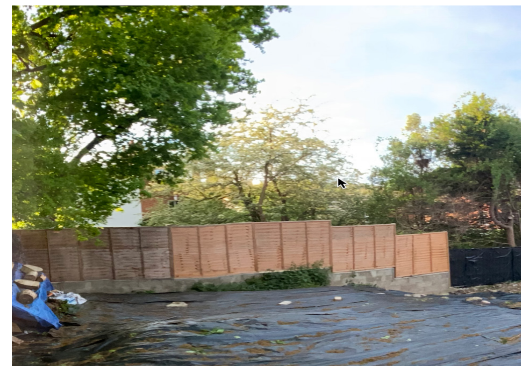
20. VIEW NORTH TOWARDS GLASSLYN ROAD FROM SEMI-DETACHED MASTER BEDROOM
