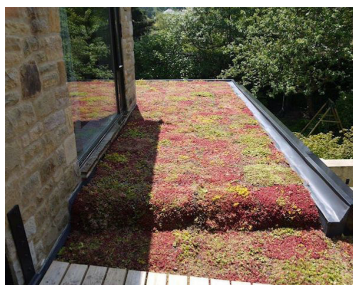
41. EXTENSIVE GREEN ROOF
