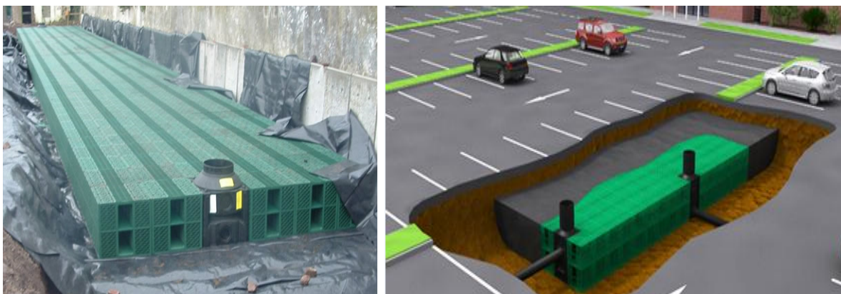
Figure 3: Typical Cellular Attenuation Tank (Hydro Stormbloc)
