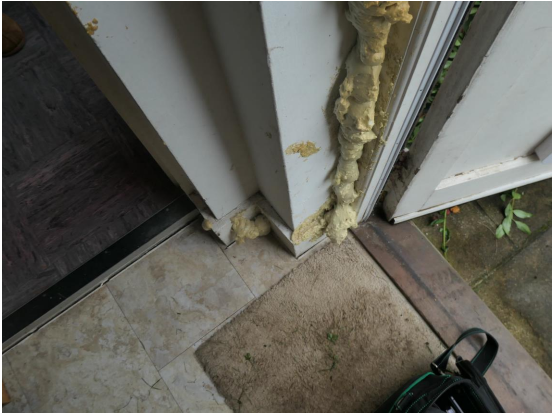
Foam into open joint now formed where extension abuts the house
