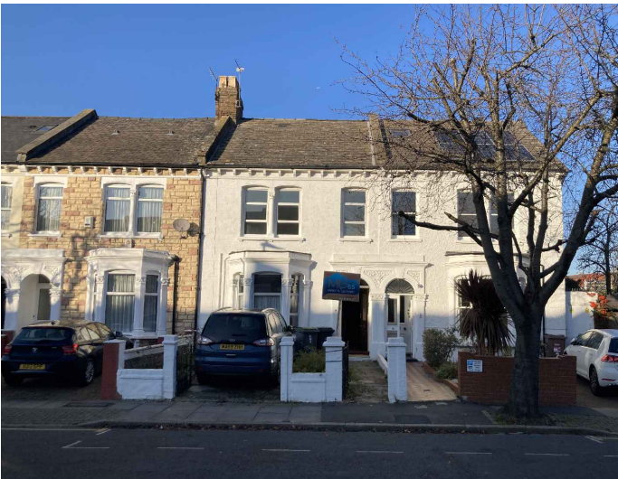
Photo 1: Existing front elevation
