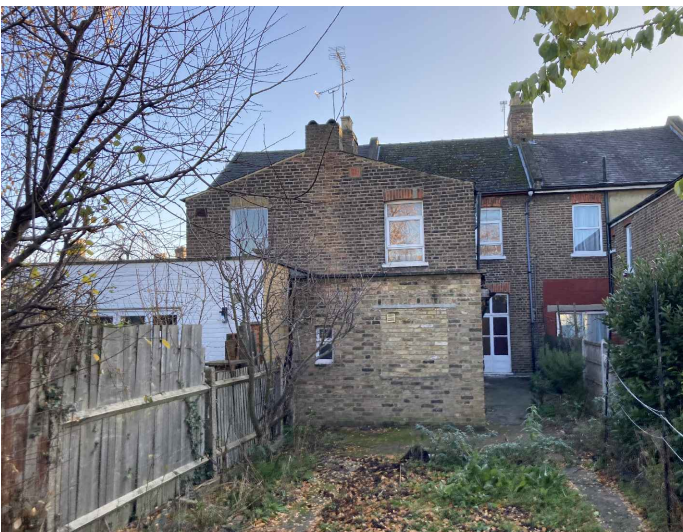
Photo 3: Existing rear elevation from garden
