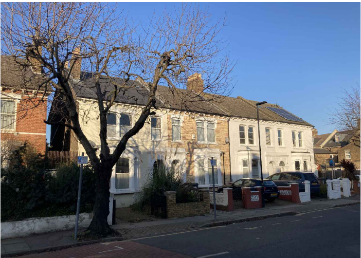
Photo 2: Adjoining neighbouring properties
