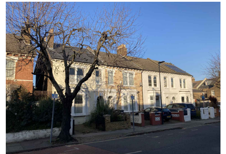
Photo 2: Adjoining neighbouring properties
