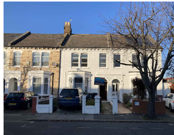
Photo 1: Existing front elevation
