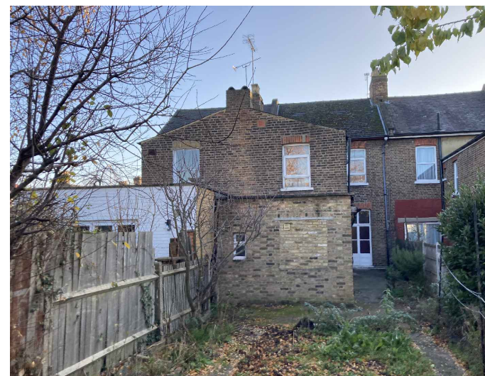
Photo 3: Existing rear elevation from garden
