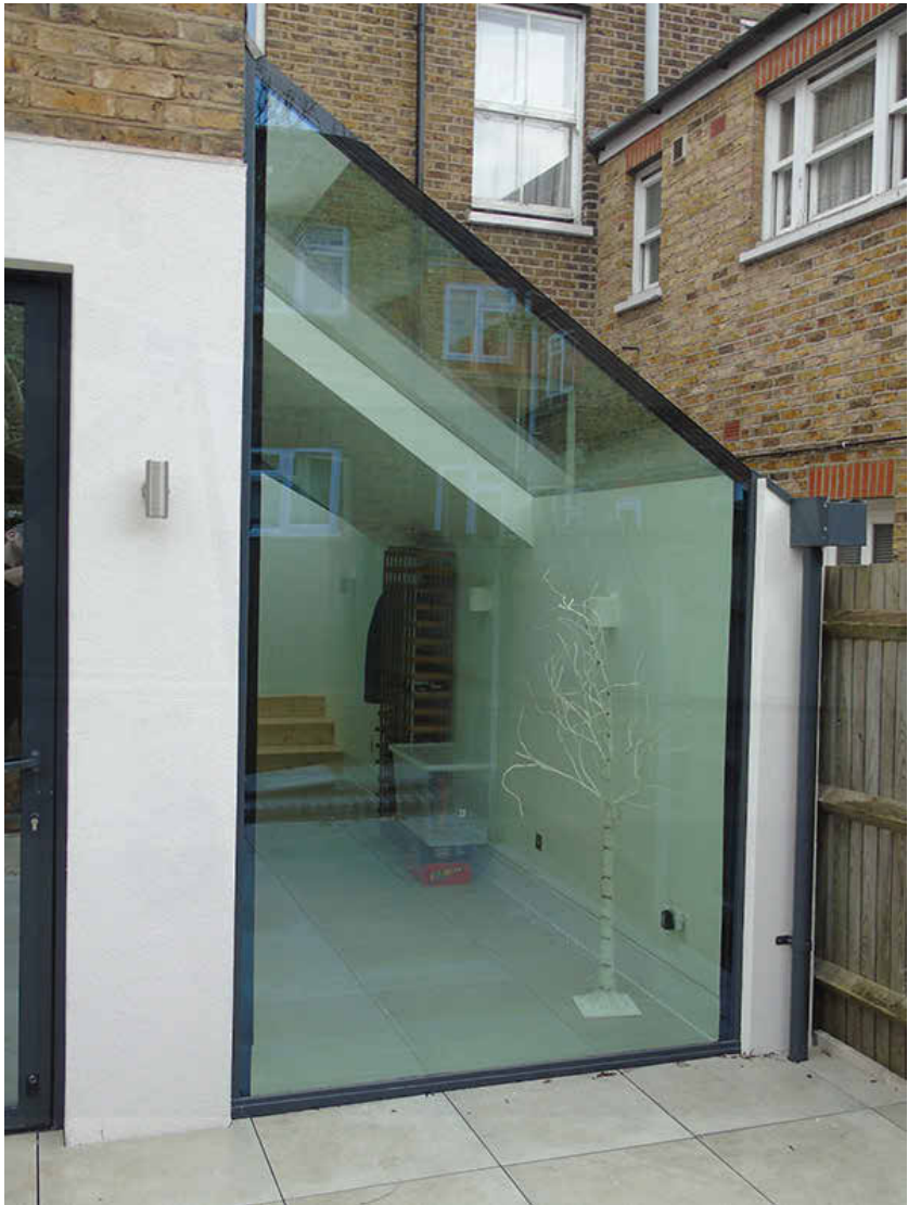
Glass pitche roof and wall examples
