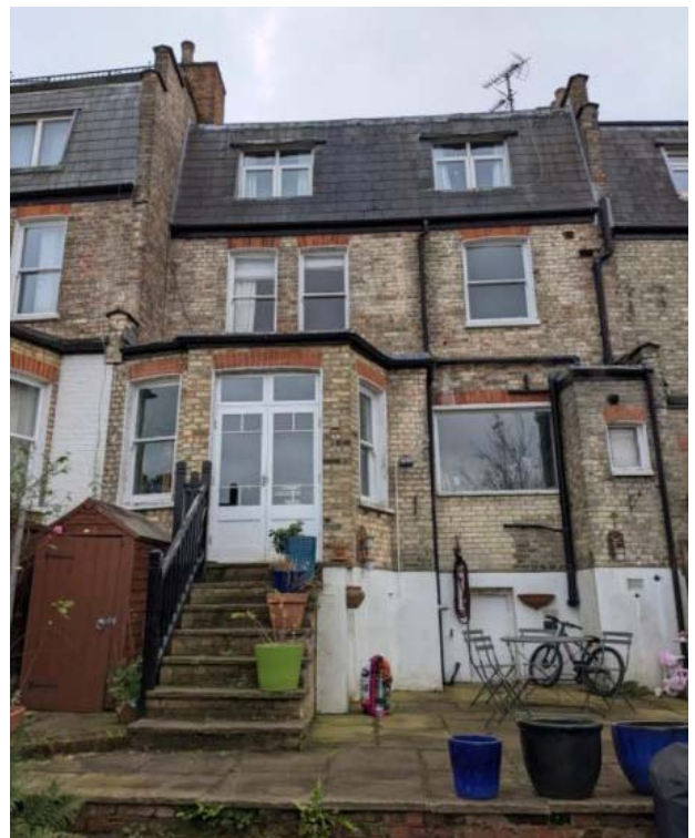
Image 05 – View of the existing rear facade of the project 1.0
