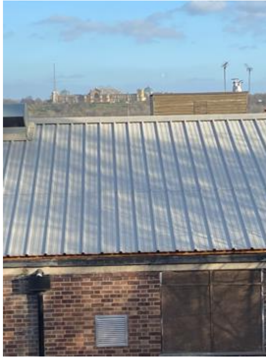
Fig. 3: Photo from existing roof terrace showing uninterrupted views to Alexandra Palace
