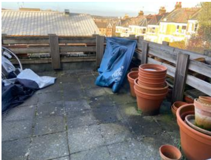
Fig. 2 Photo showing existing first floor roof terrace
