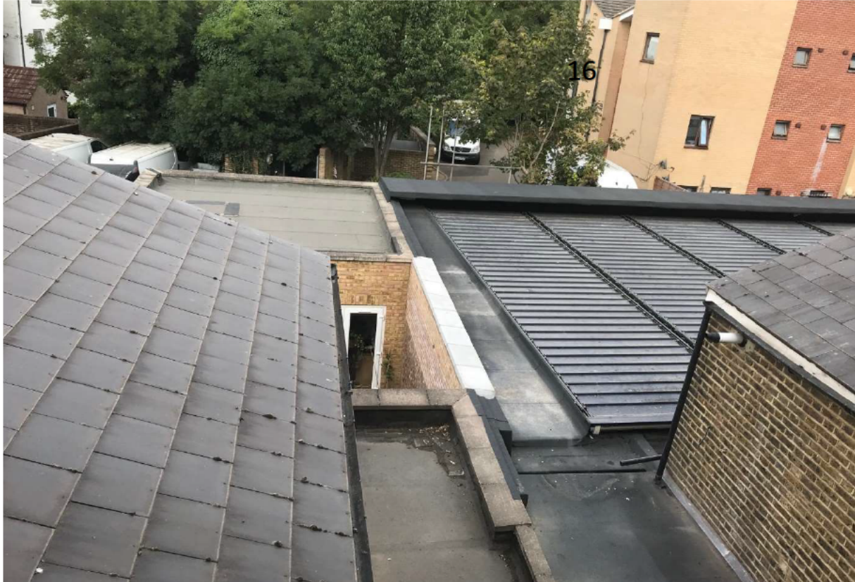
Fig 03: The rear view from first floor window of Flat 2
