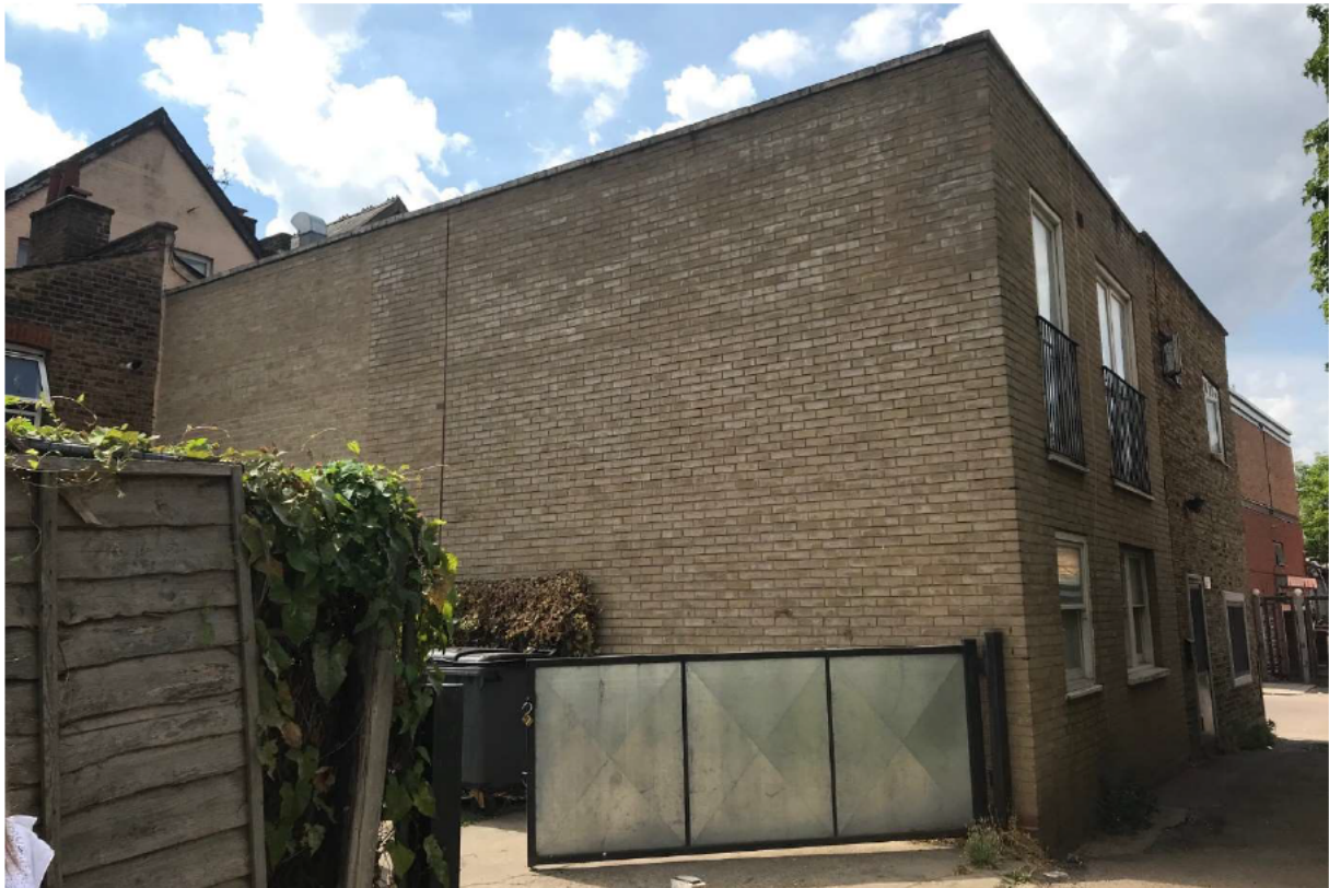
Fig 08: The rear view, neighboring double storey extensions. No. 468 & No.470 West Green Rd
