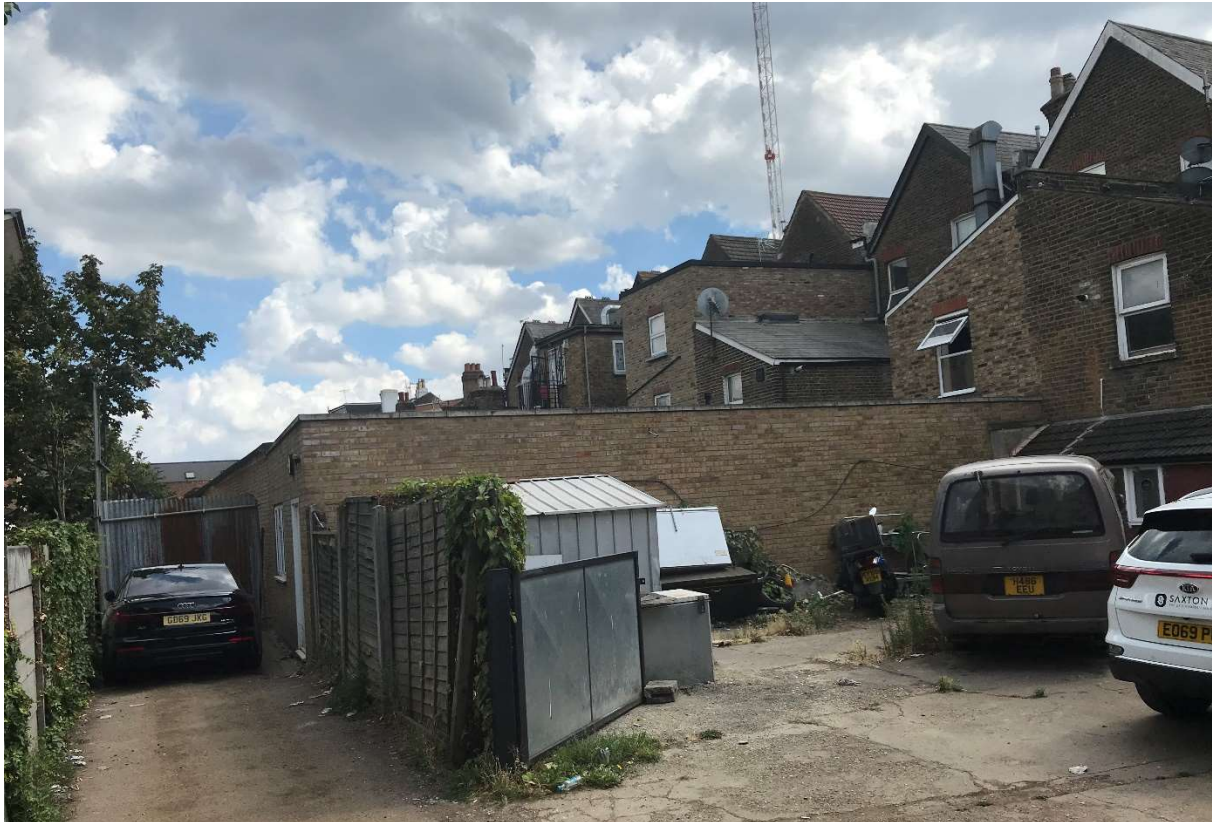
Fig 02: The rear view from roadway, existing single storey extension
