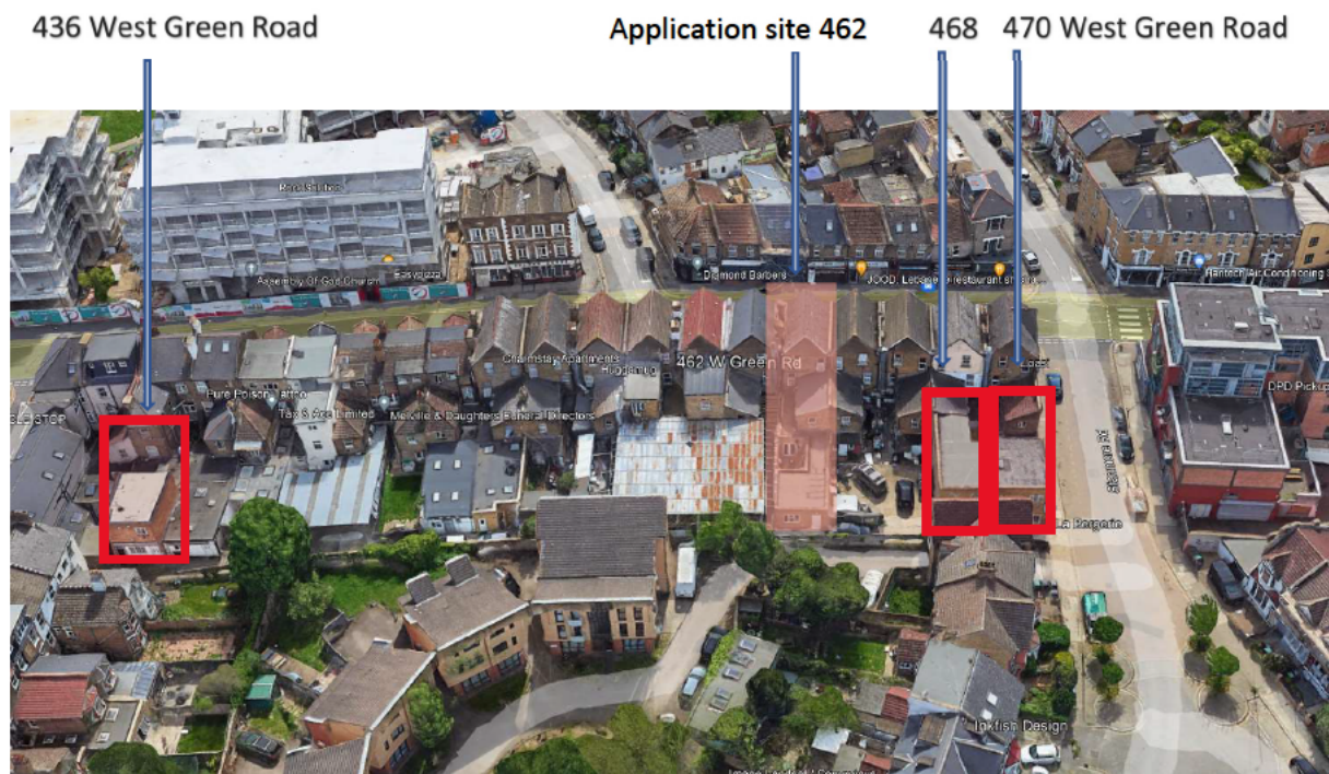
Fig 09: The rear view, Double storey extensions. No. 436, 468 & No.470 West Green Rd
