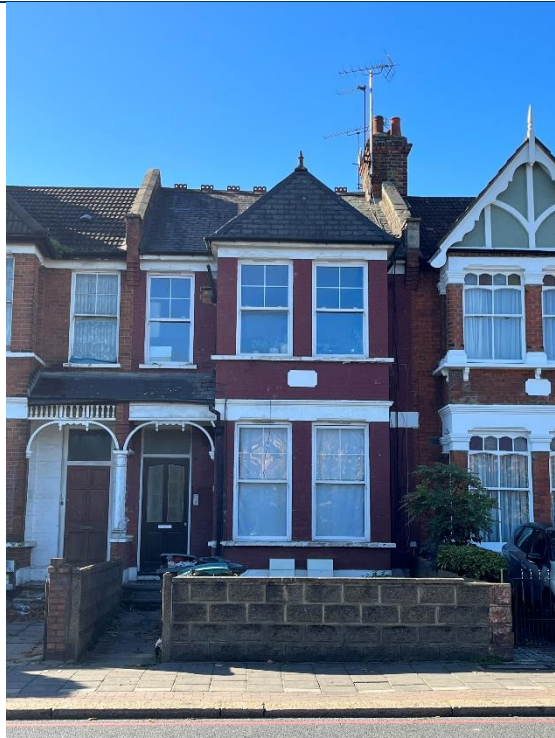
Photo 01 Existing Front Elevation
