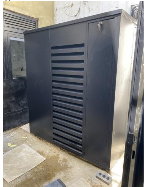
Figure 1– Typical Condenser Attenuated Enclosure
