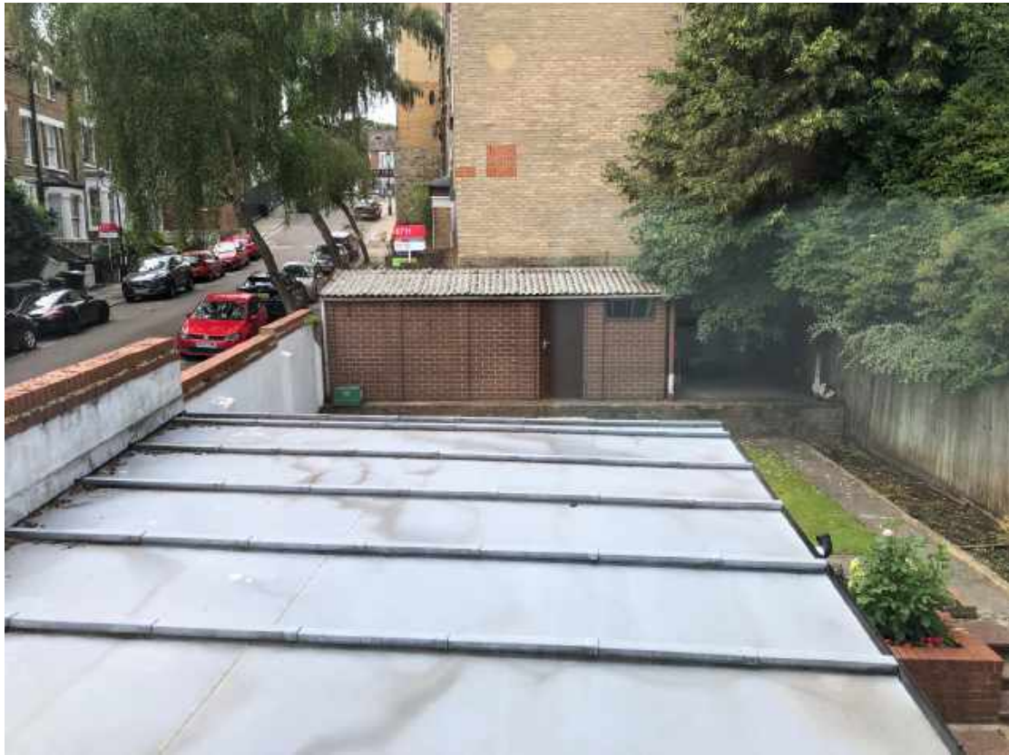
View from first floor of house over single storey rear extension towards rear of site containing stepped garden, garage building, lime tree and flank wall of no.11 Wembury Road
