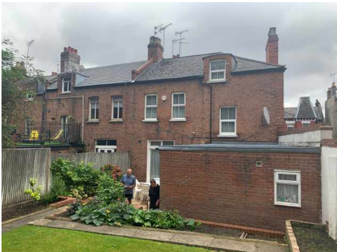
View of rear of house and single storey rear extension from garden
