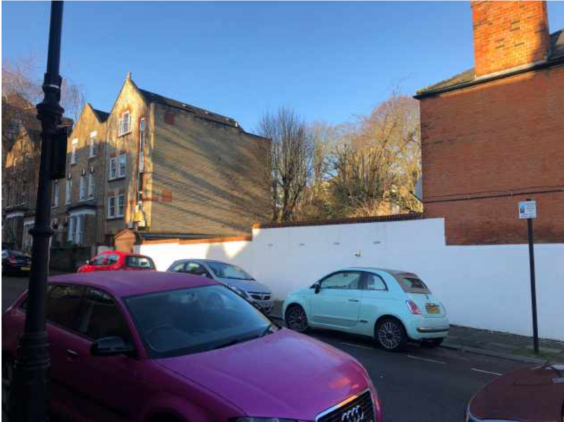
Street view of boundary wall of rear of site on Wembury Road with flank wall of no.41 Langdon Park Road on right and no.11 Womersley Road on left
