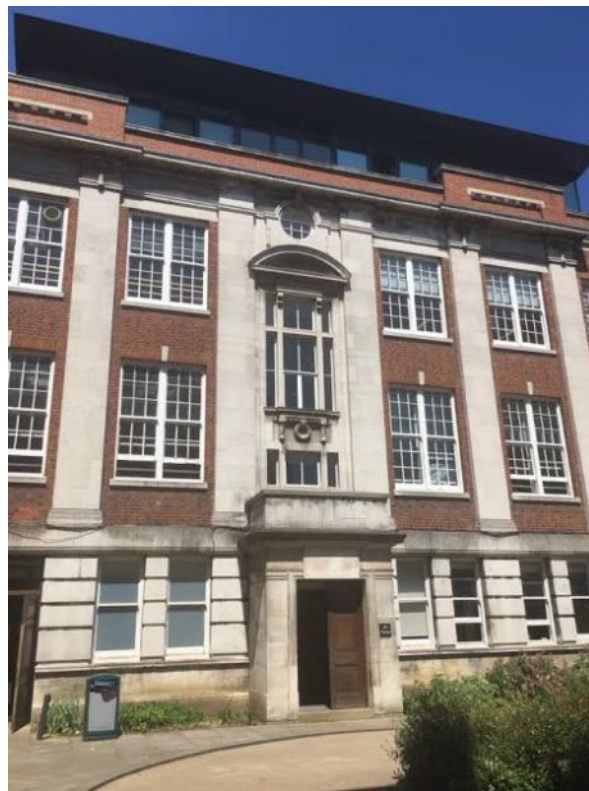
Figure 71. Southern façade to Science Quad.
