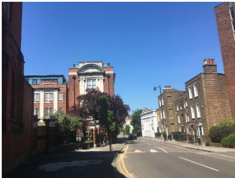
Figure 125. View Southwood Lane seen adjacent to the flank elevation of the Big School.
