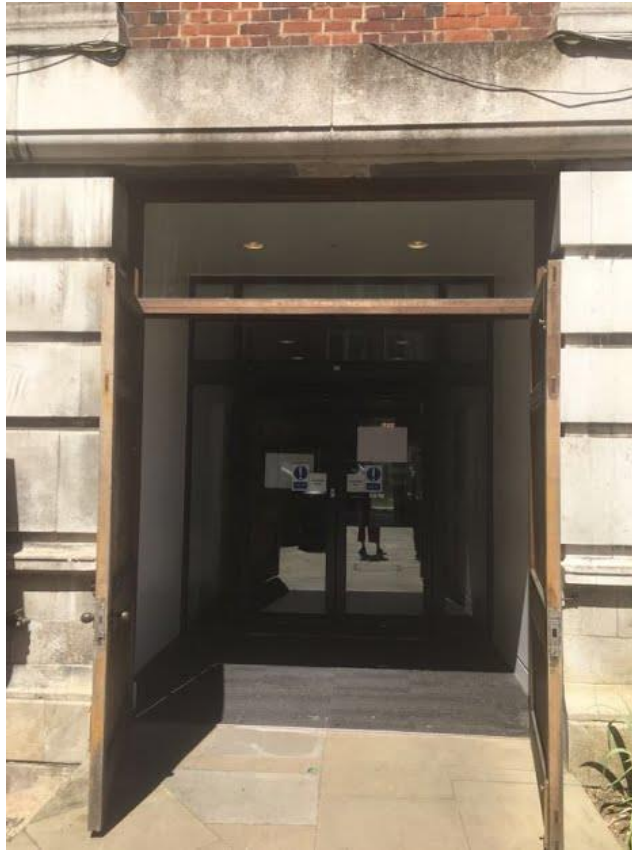
Figure 81. Modern sliding door within new linking corridor between Science Quad and Garner Building.
