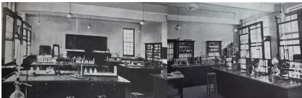
Figure 25. The 'Elementary' and 'Advanced' Chemistry Labs at second floor within the North Road wing. Note specialised window casements, creating fume cupboards.
