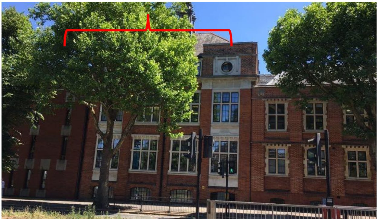
Figure 127. View east towards the North Road façade of the Science Building. Extent of the façade indicated by the red bracket.
