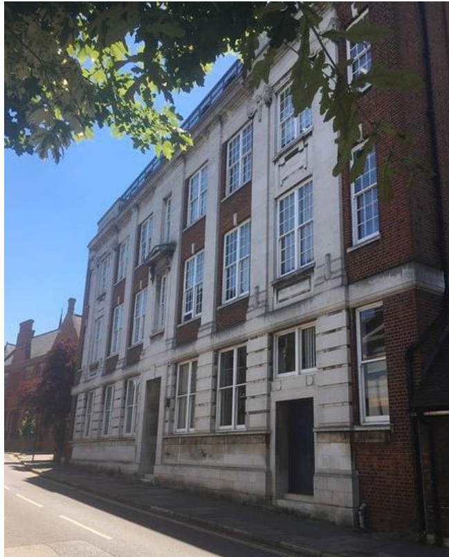
Figure 70. Southwood Lane façade, note two blocked entrance doors.
