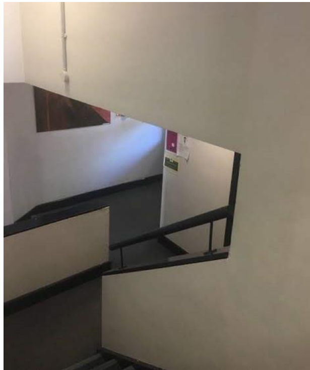
Figure 77. Modern stair leading to Garner Wing.
