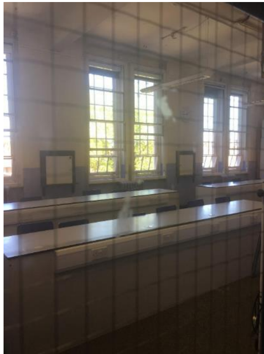
Figure 99. Note secondary glazing and modern fit out to interior including suspended strip lighting.
