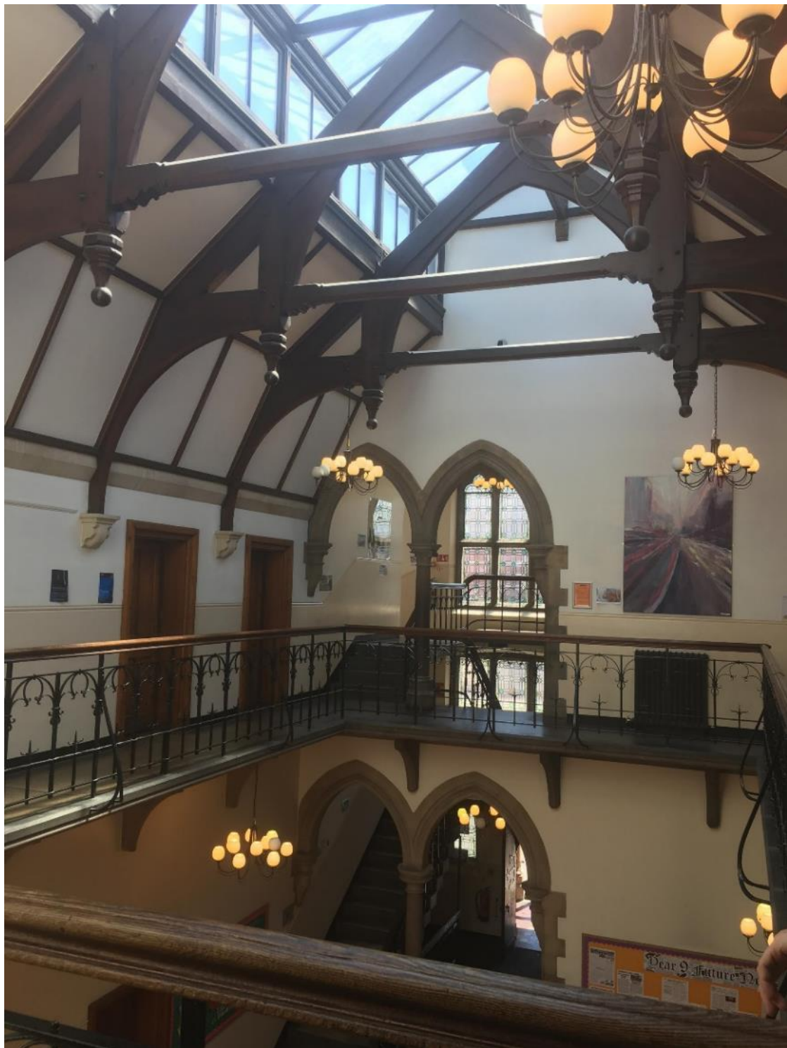
Figure 118. Central hall, note gothic detailing including pointed arches, stone mullions to windows and tri-foil ironmongery to balustrade.
