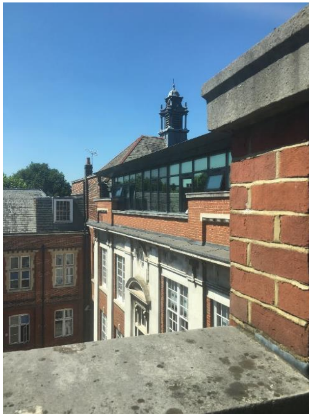
Figure 114. View of existing parapet looking north west toward cupola.
