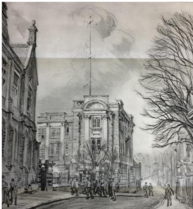
Figure 35. Science Building, 1959. Note structure above east-west wing seen centrally and exposed parapet level to Southwood Lane.
