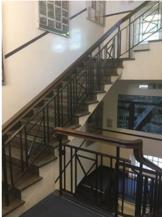
Figure 103. Note geometric pattern to balustrade ironmongery repeated within Science Quad railings.
