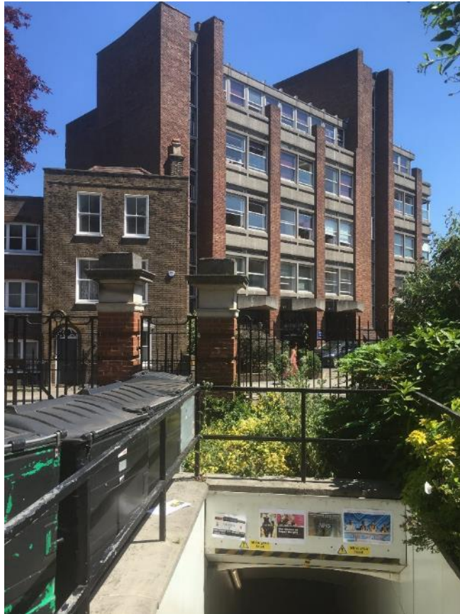
Figure 73. Tunnel to Dyner building from Science Quad.
