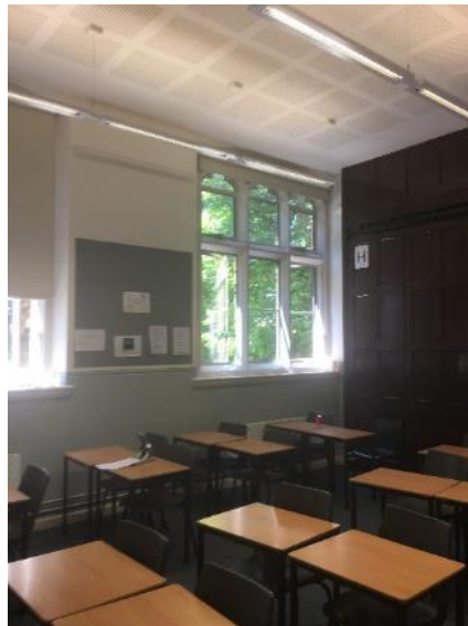
Figure 119. Timber panelling and tri-foil stone carving to window reveal within central hall classroom.
