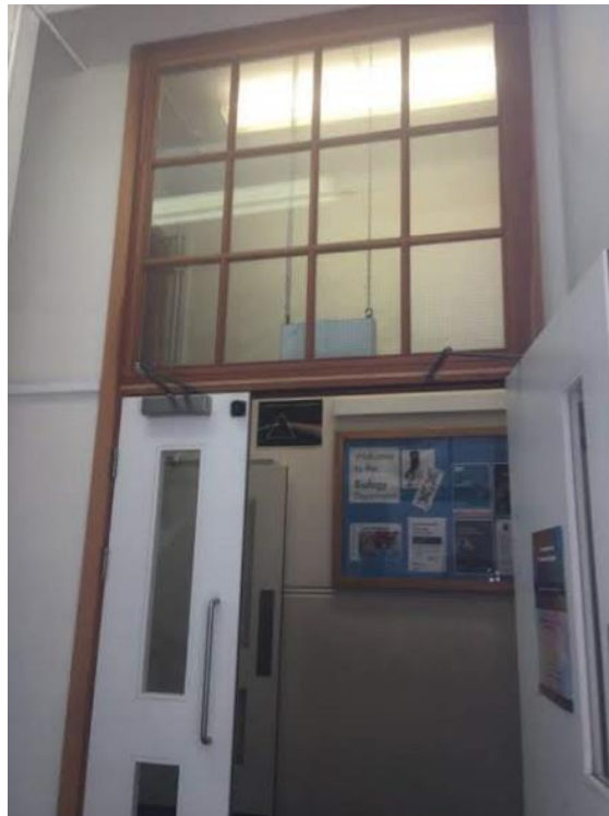
Figure 85. Modern fire-door within internal corridor of Science Building.
