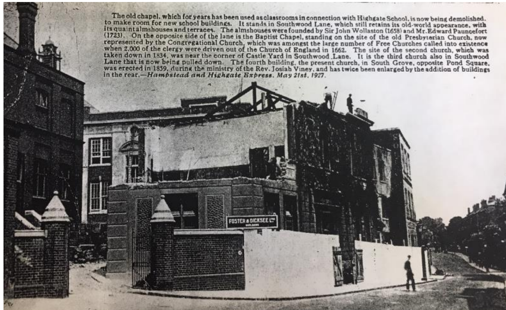
Figure 16. Demolition of the old chapel buildings to create the new Science Building, under conduction in this image.
