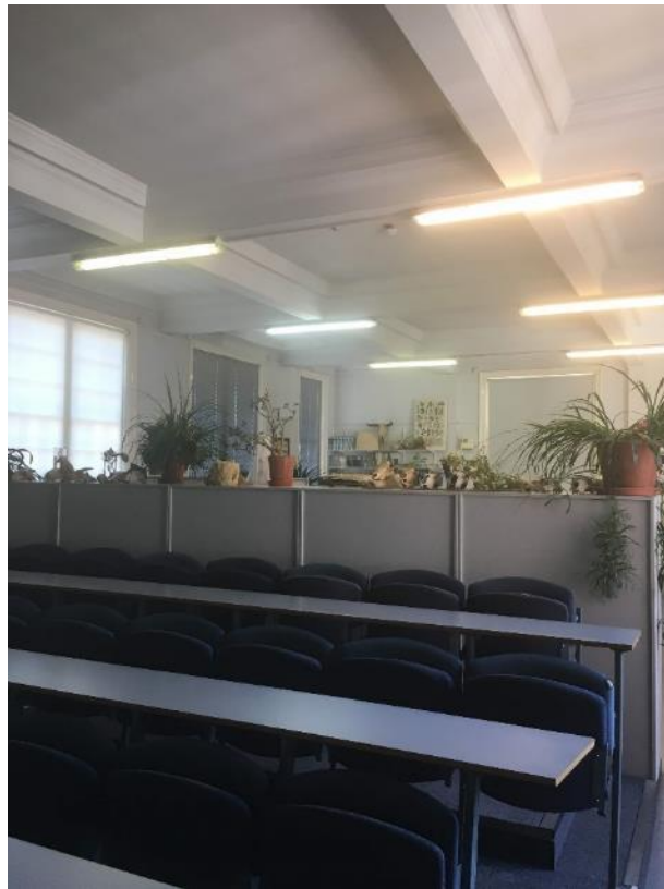
Figure 108. Note cross beams to ceiling and retained lecture-seating, albeit with modern fixture and fittings.
