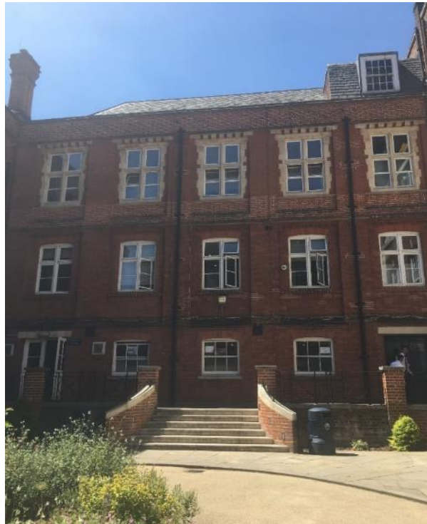
Figure 82. Northern elevation of nineteenth century central hall block opposite the Science Building.
