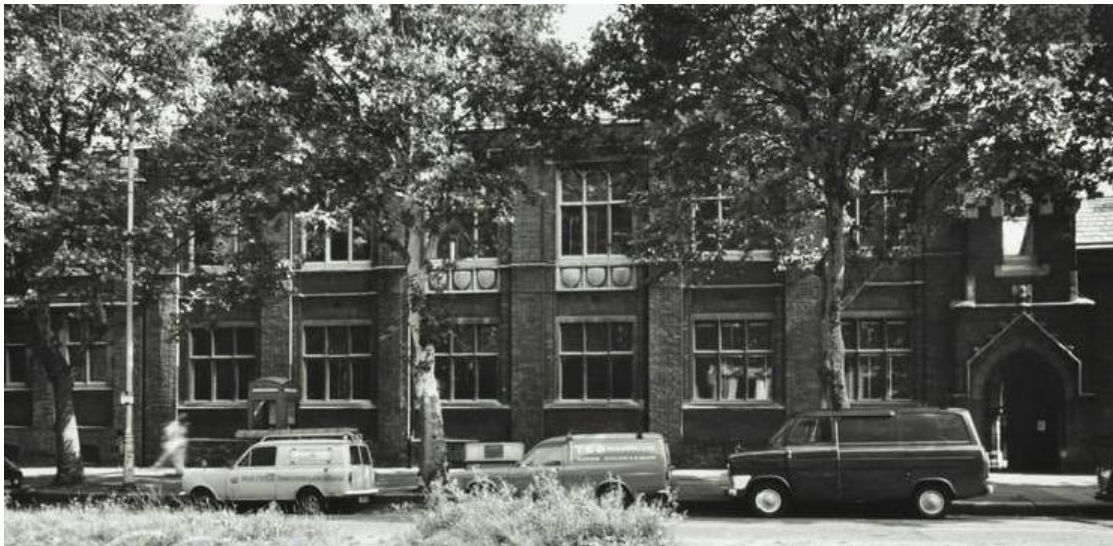
Figure 47. Highgate School North Road exterior, looking west towards 1890s extension, c. 1980.
