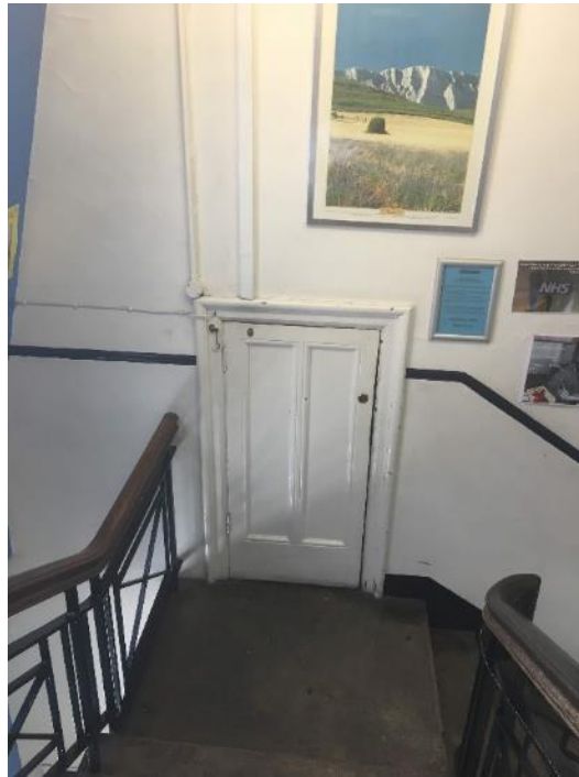
Figure 115. Doorway at landing, connecting Science Building to adjacent central hall.
