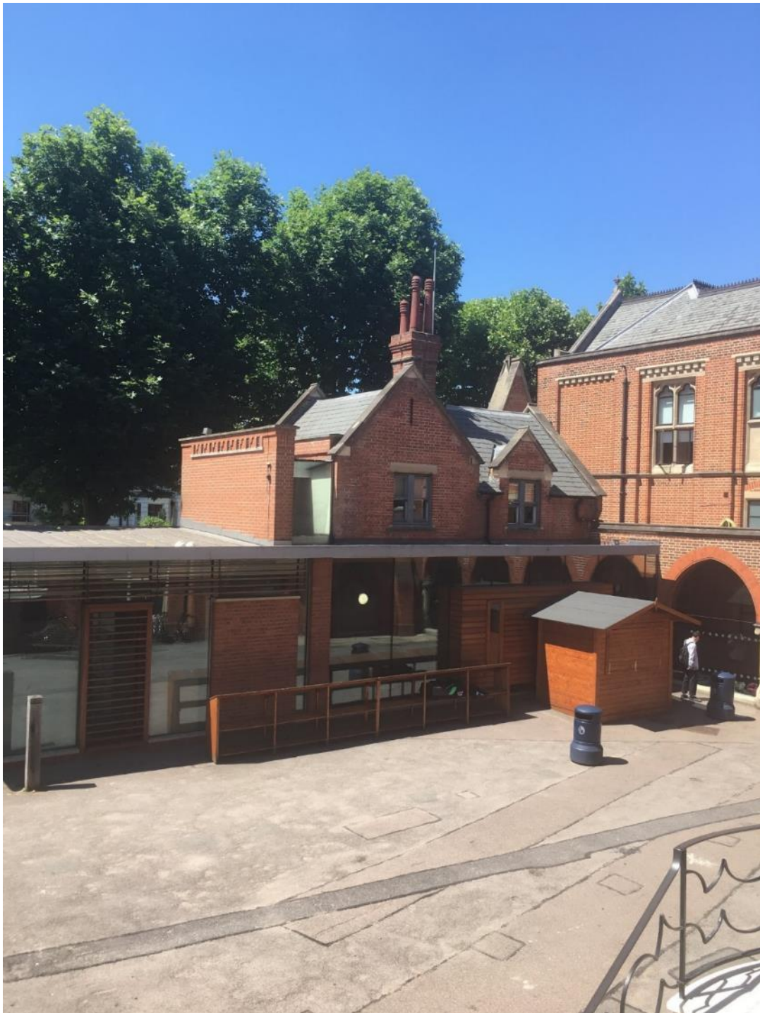
Figure 122. Modern reception extension to North Road
