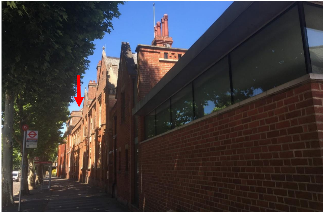
Figure 126. View north along North Road adjacent to the modern extension to the entrance lodge. The flank elevation of the Science Building is easily distinguishable through the rise in the parapet level and change in aesthetic. This image shows the considerable variety of style and age to the built fabric along North Road, including several contemporary and late twentieth century additions. The location of the Science Building is indicated by the red arrow.
