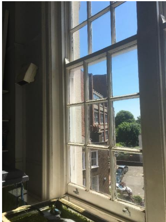
Figure 110. Detailed view of original nine over nine sash window with timber frame.
