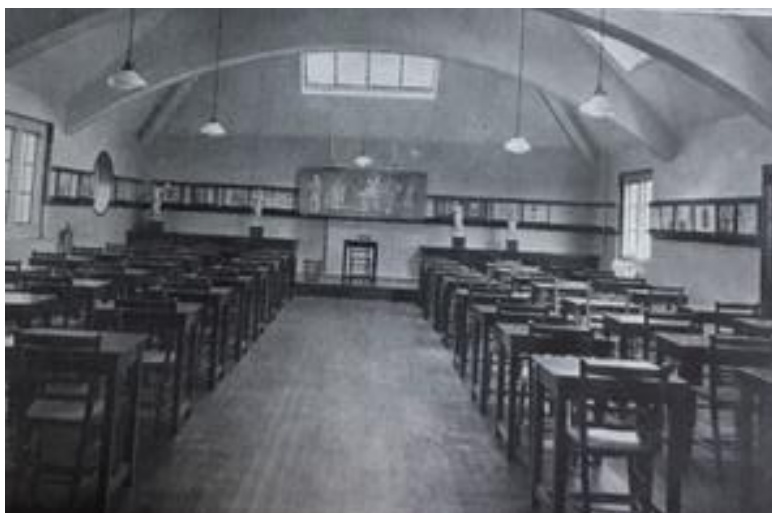
Figure 27. The Art School at third floor to North Road, note round window and curved support beams to roof.
