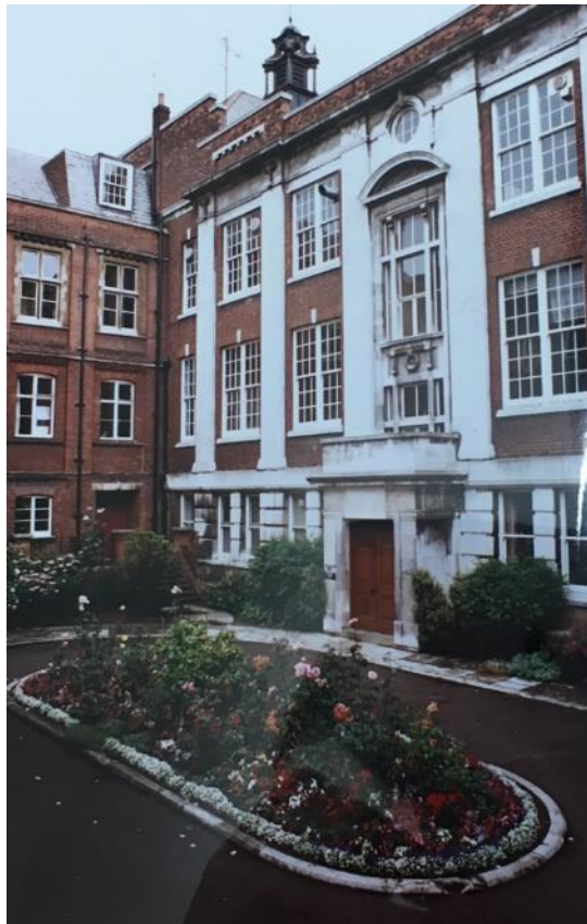
Figure 42. External façade of Science Building Seen from the courtyard, c. 1980.
