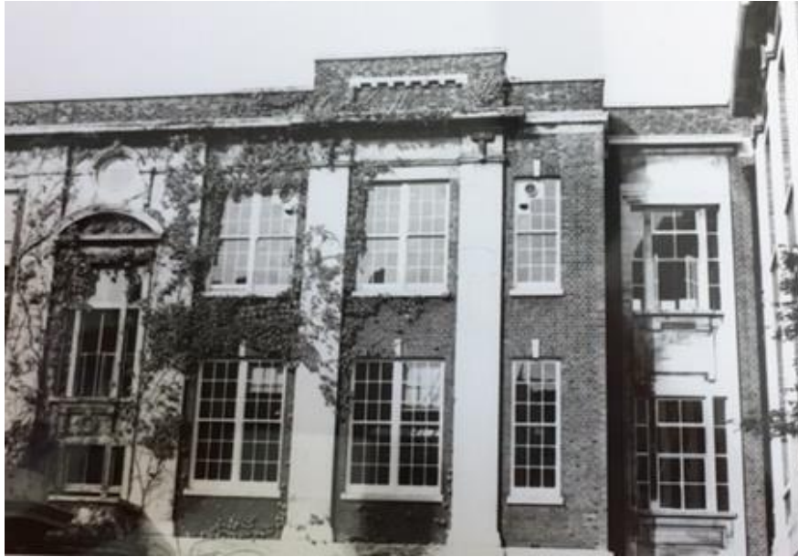
Figure 32. View within Science Building Courtyard, circa 1940s. Note change in fenestration within entrance bay to the right of the image and above entrance bay to the left.
