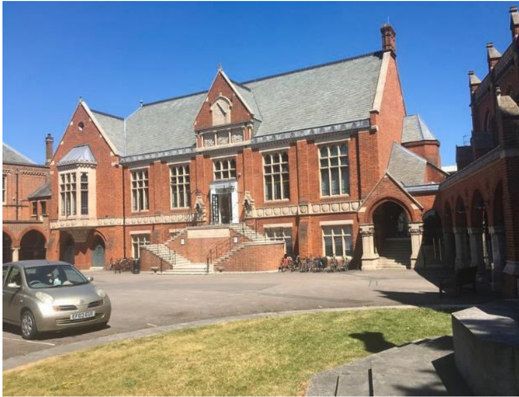
Figure 123. 'Big School' or the 'Old School Building' Grade II, to the south of the site seen from North Road. The Chapel is visible to the right and the 1890s extension just visible to the left. The steps are a later addition, added as a memorial post 1945.
