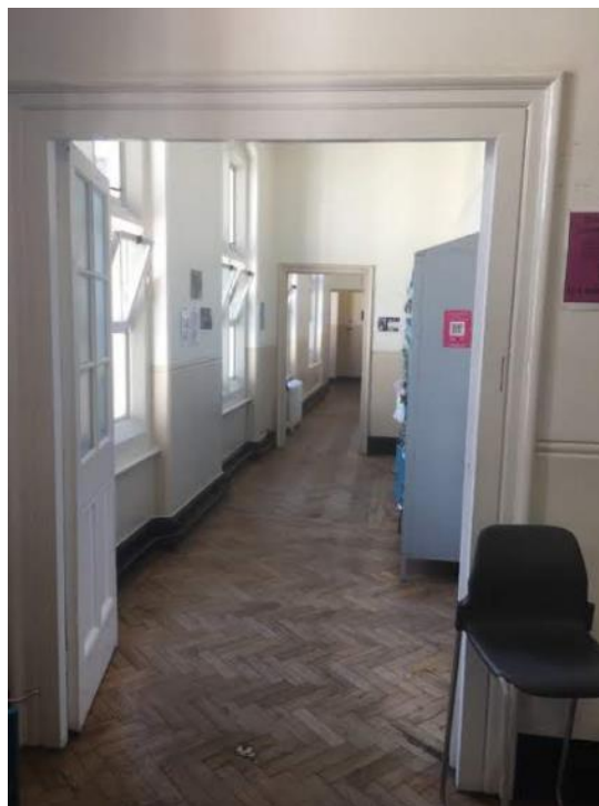
Figure 116. Connecting corridor leading from Science Building to adjacent central hall.
