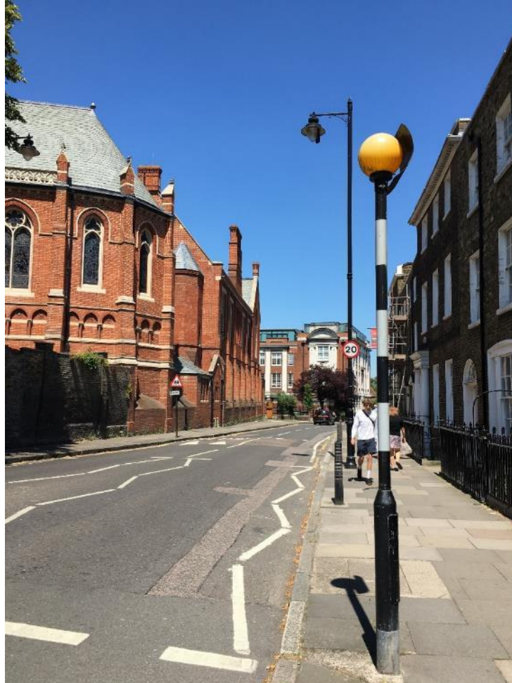
Figure 60. Distant view of Science Building from Southwood Lane. Note the clearly visible roof extension and lack of a balanced formal façade when viewed from this direction.
