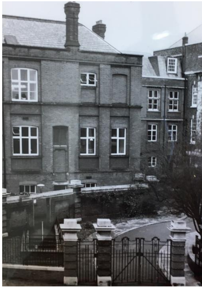
Figure 34. View within Science Building Courtyard looking south towards Central Hall flank elevation. C. 1950.
