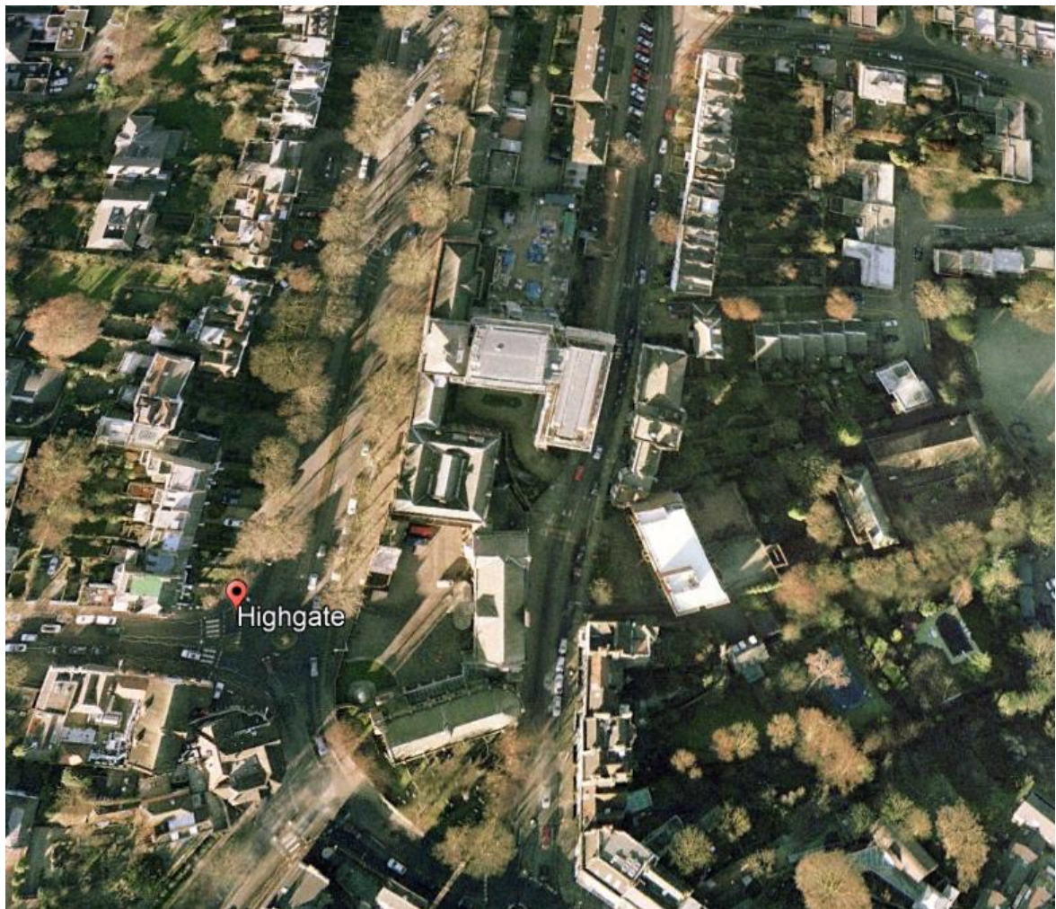
Figure 58. Aerial photo 2006. This map shows the roof extension to the Science Building, added in 2004
