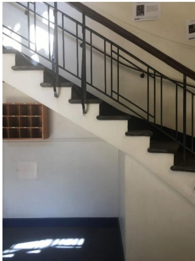
Figure 84. Originally ironmongery to balustrade within stair to the north-south wing.
