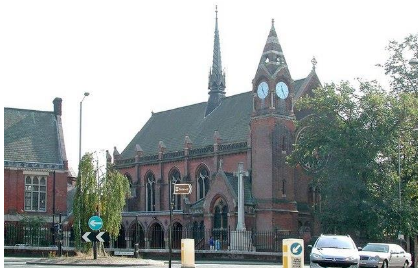
Figure 124. Highgate School Chapel, seen from the north west.
