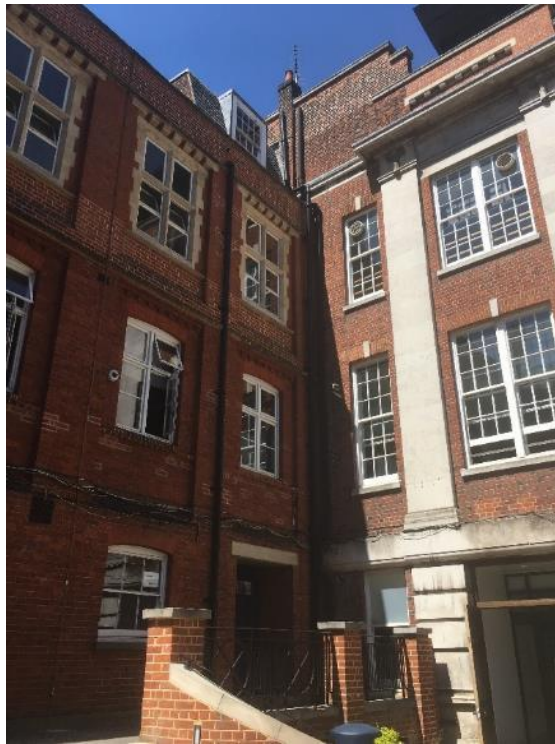
Figure 83. Connection between central hall and the Science Building, note modern alterations at ground floor.
