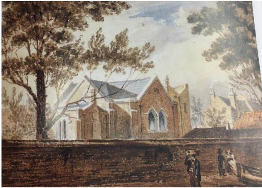
Figure 5. The Old School in 1833 viewed from Southwood Lane following the demolition of the chapel and prior to the extension works of 1845.
