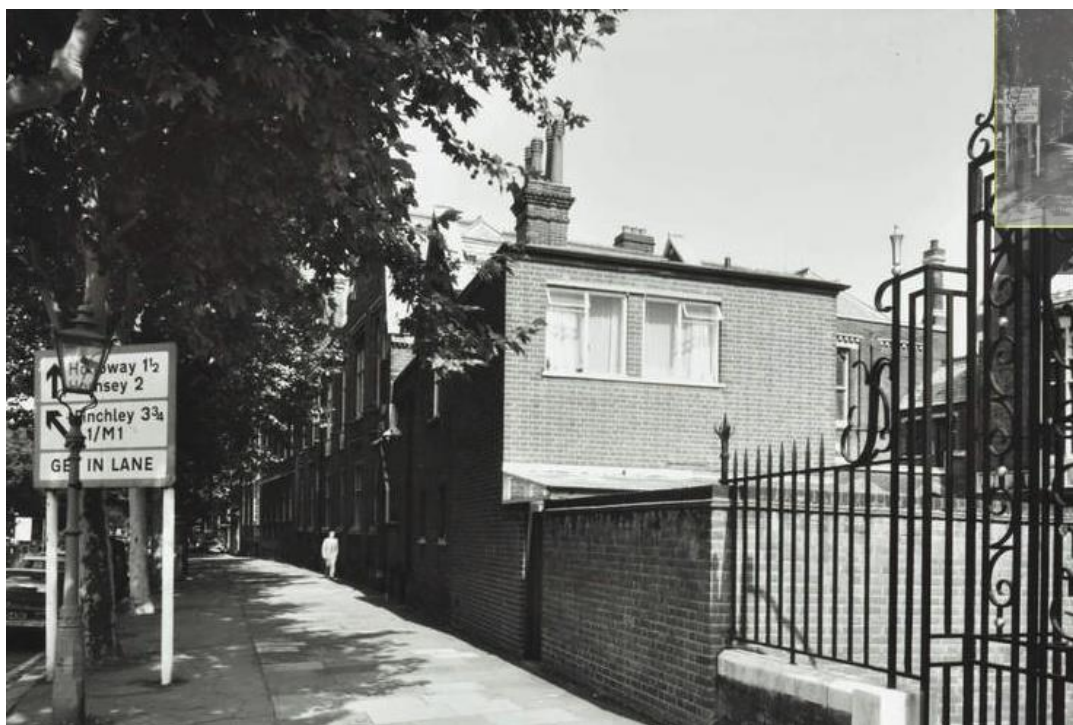
Figure 45. Highgate School North Road exterior, looking north west, c. 1980.
