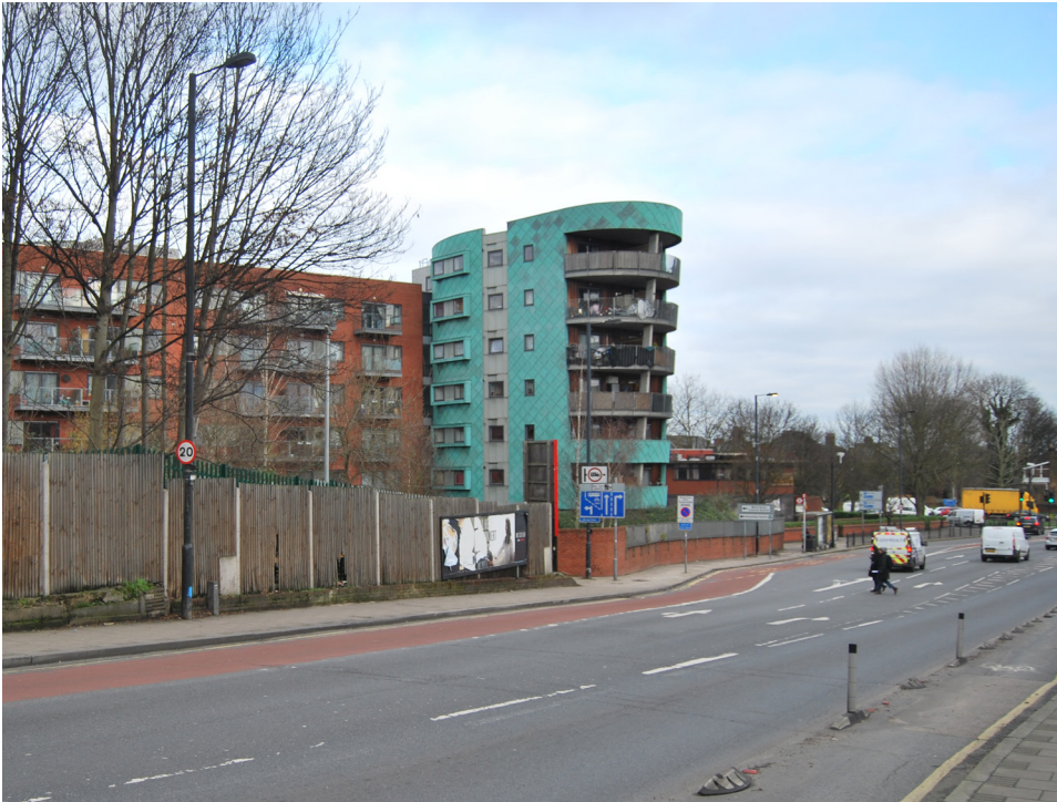
VIEW 2 LOOKING EAST FROM TURNPIKE LANE
