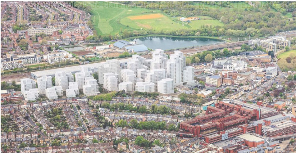
GAS WORKS MASTERPLAN UNDER CONSTRUCTION
