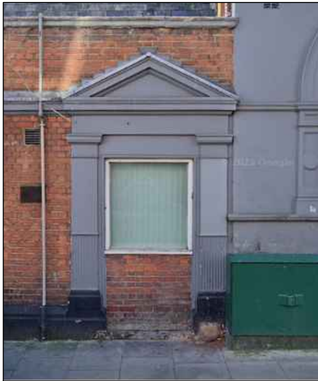
EXISTING WINDOW OPENING
