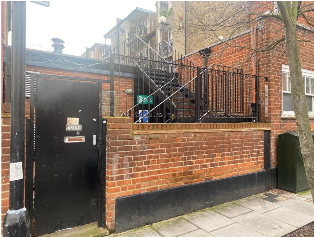
Access to the staircase from the street
