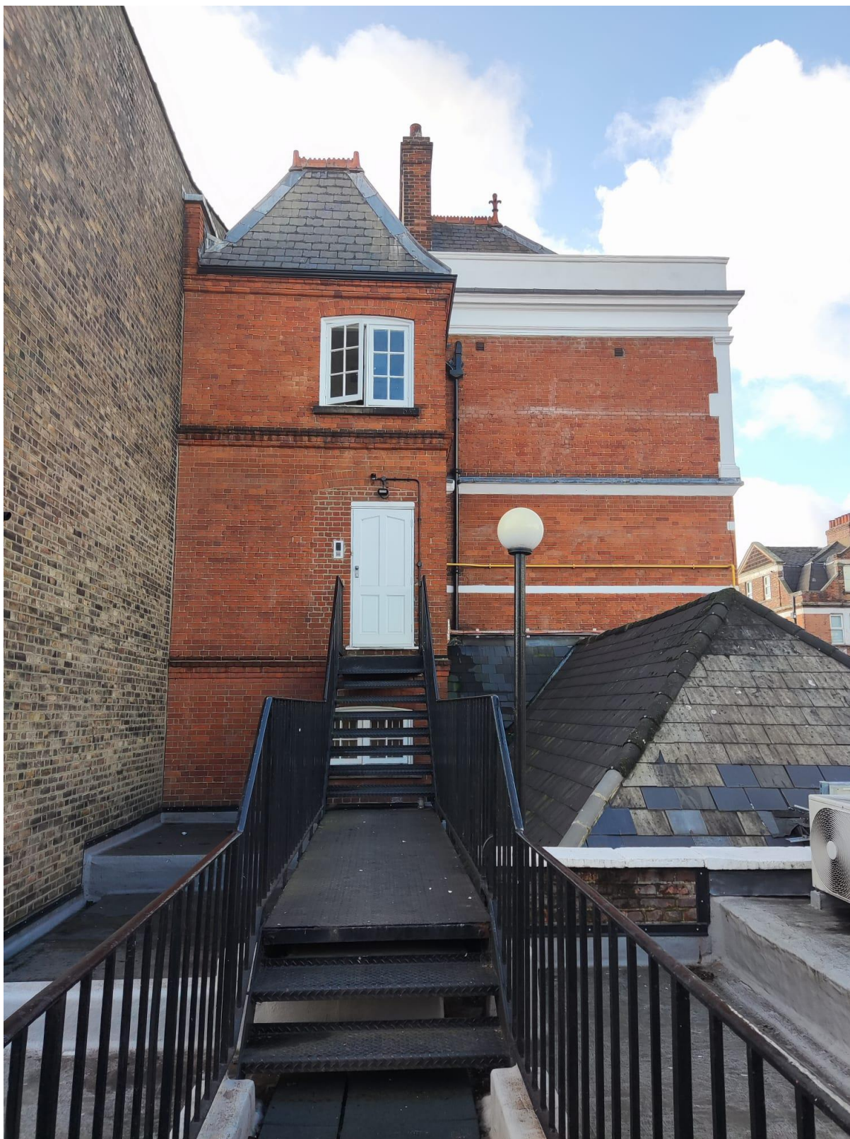
The doorway at the end of the access walkway leading to the communal staircase to the flats
