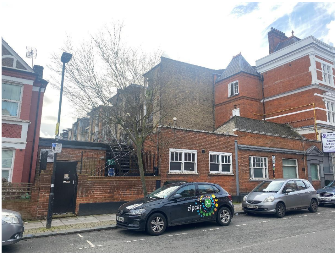
Views from Stanhope Gardens with the current entrance at the rear
