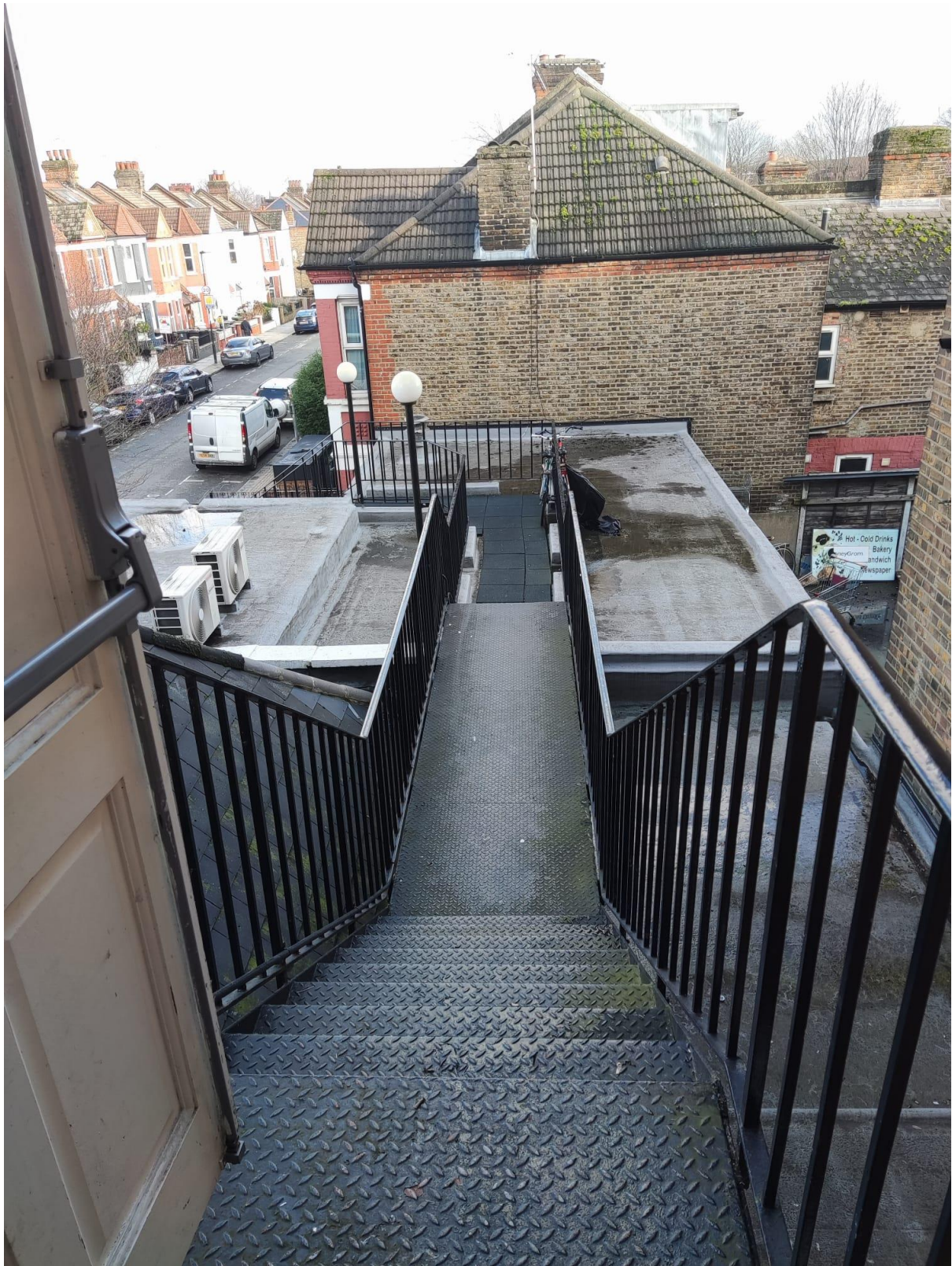
The access walkway over the flat roof leading to the flats
