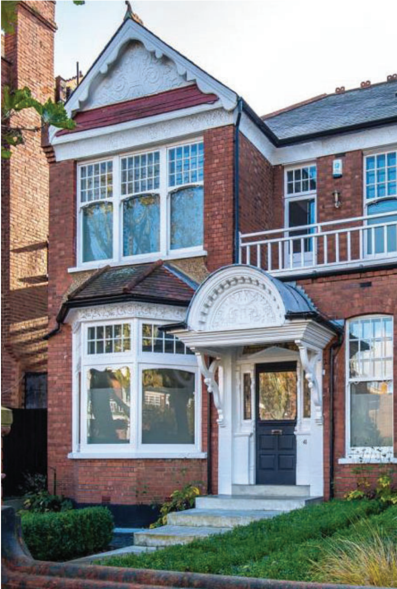
EXISTING FRONT ELEVATION - BAY WINDOW AND ENTRANCE
