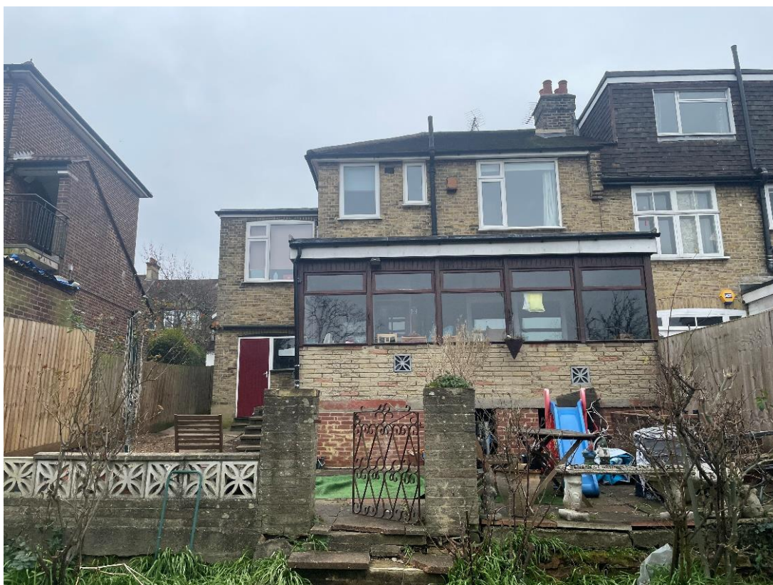
Rear elevation – February '23
