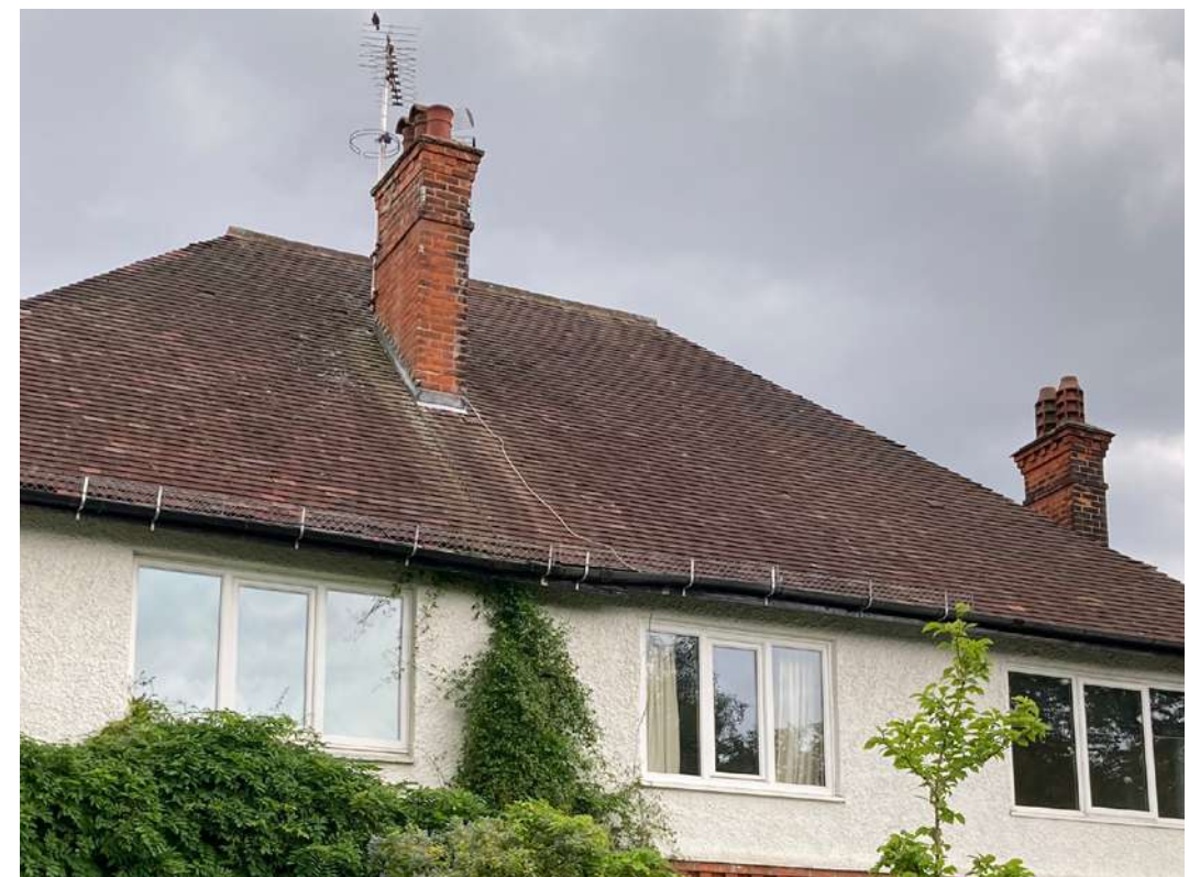
Existing roof - rear view
