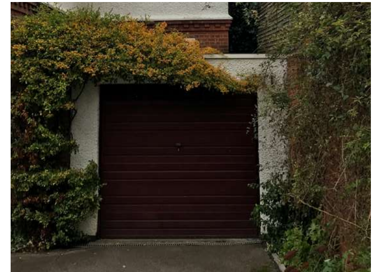
View of no. 11A garage added in the 1960s
