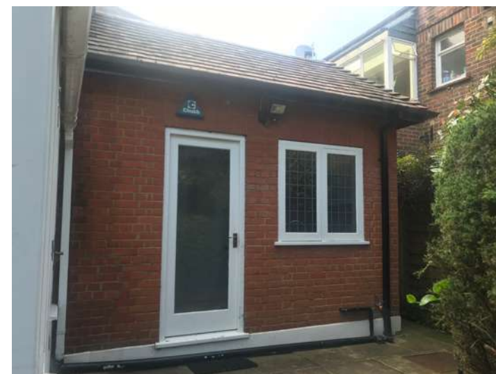
No. 11 garage - rear view
