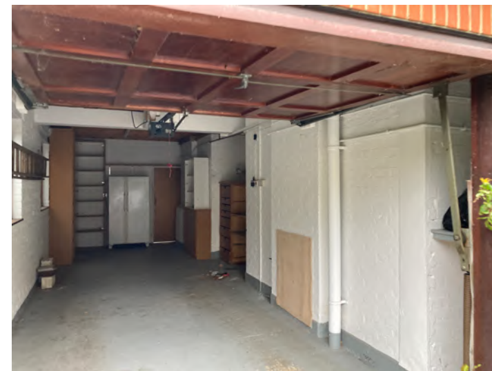
No. 11 garage interiors
