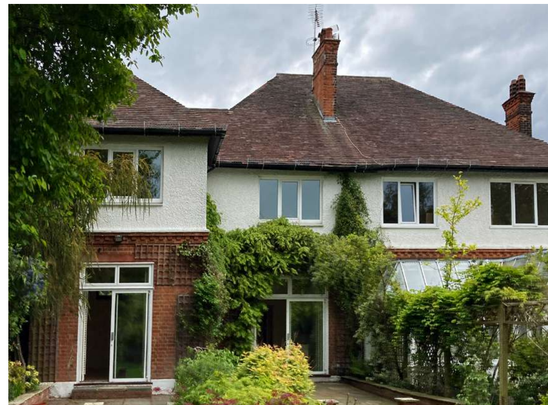
2. Rear of the house
