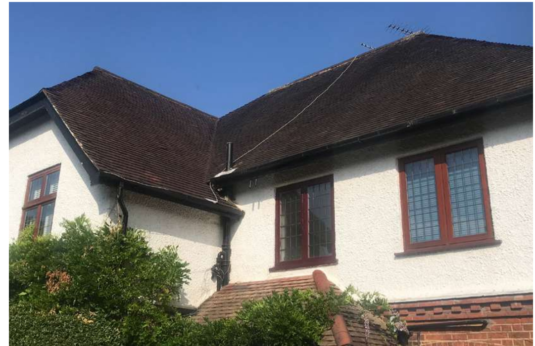
Existing roof - front view
