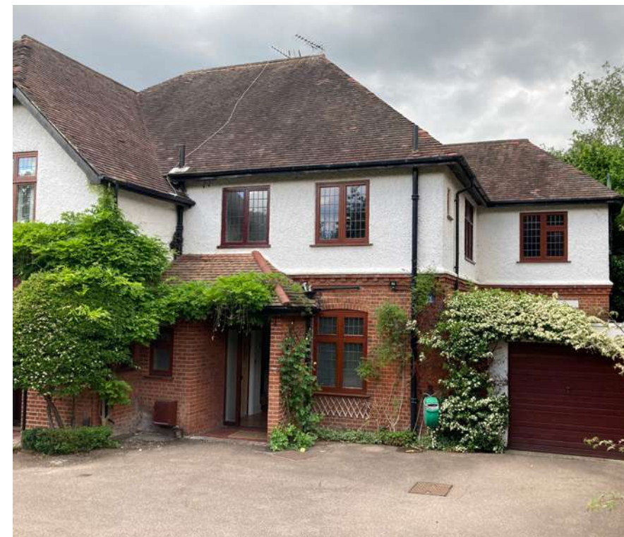
4. Access to no. 11A
