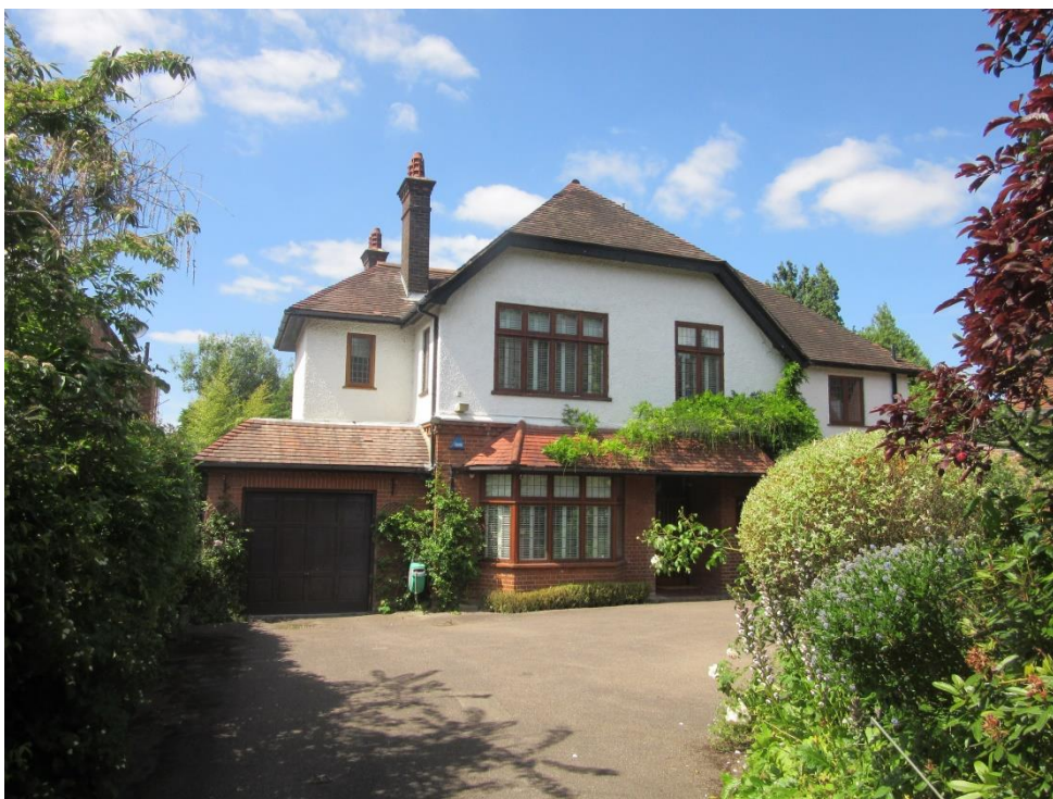
Figure 26: The front elevation of 11 View Road.
