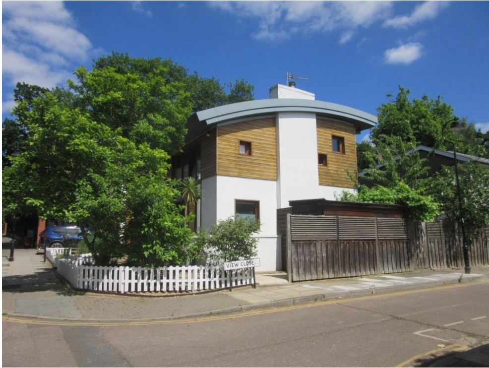
Figure 10: No. 14 View Road, built in 2006.
