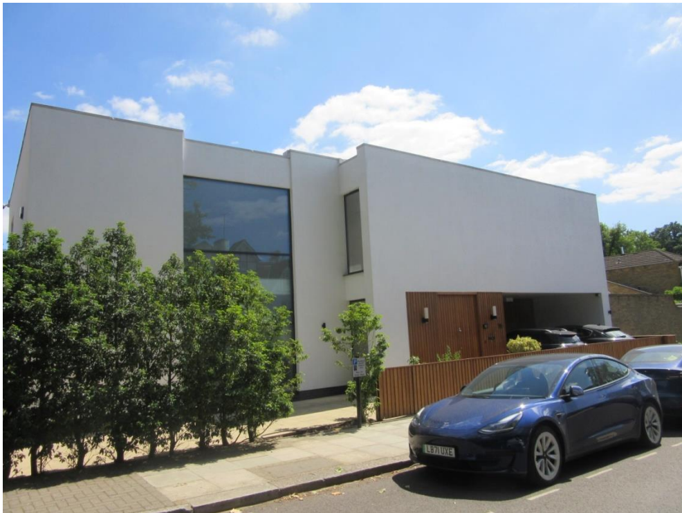
Figure 11: No. 16 View Road, built in 2010.
