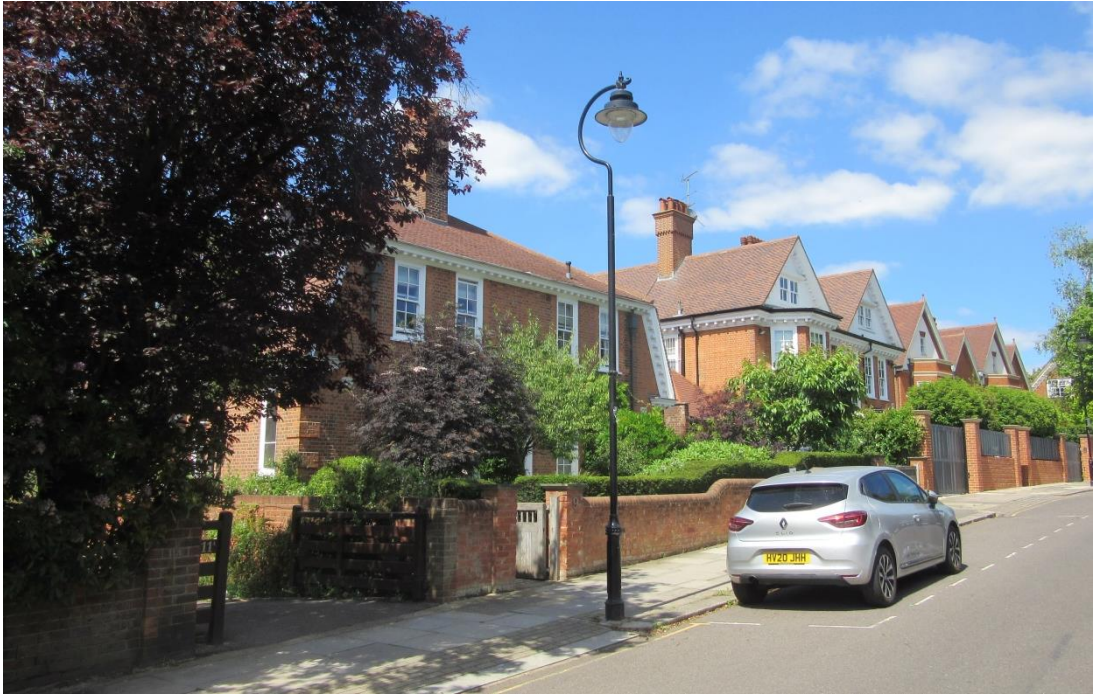
Figure 4a: The north side of View Road, with the Grade II listed No. 9 (left), locally listed No. 7 (centre) and rebuilt No. 5 (right) forming an architectural group – the driveway to the subject site is to the far left.
