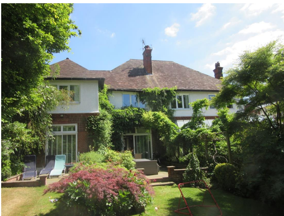
Figure 27: The rear elevation of 11a View Road.
