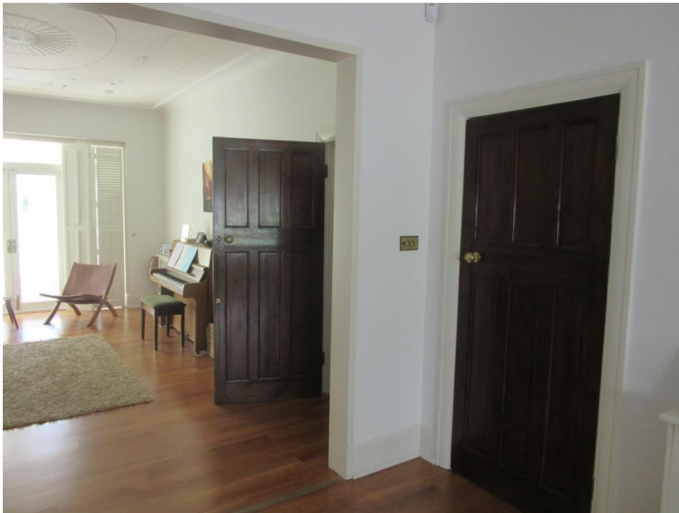
Figure 30: The principal rooms of No. 11 illustrating loss of original detailing and plan form except the doors.
