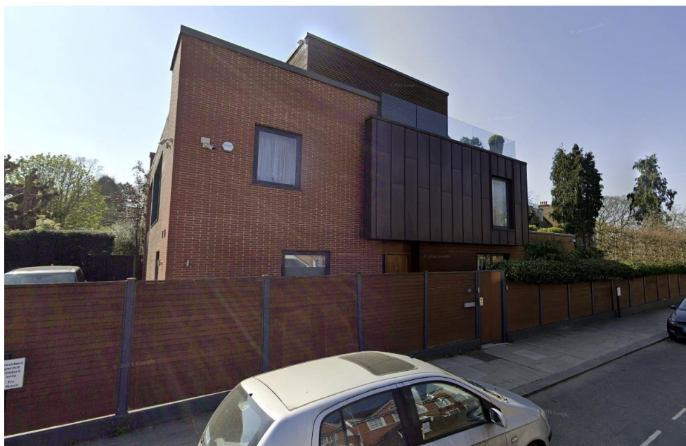
Figure 8: No. 8 View Road, built in 2006.
