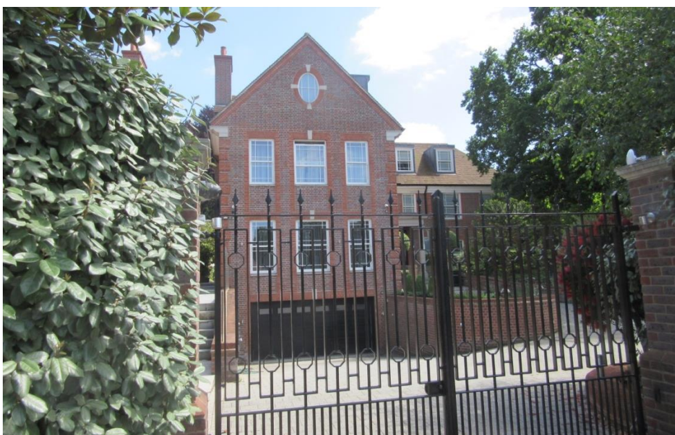
Figure 9: Nos. 10 and 10a View Road, built in 2010.
