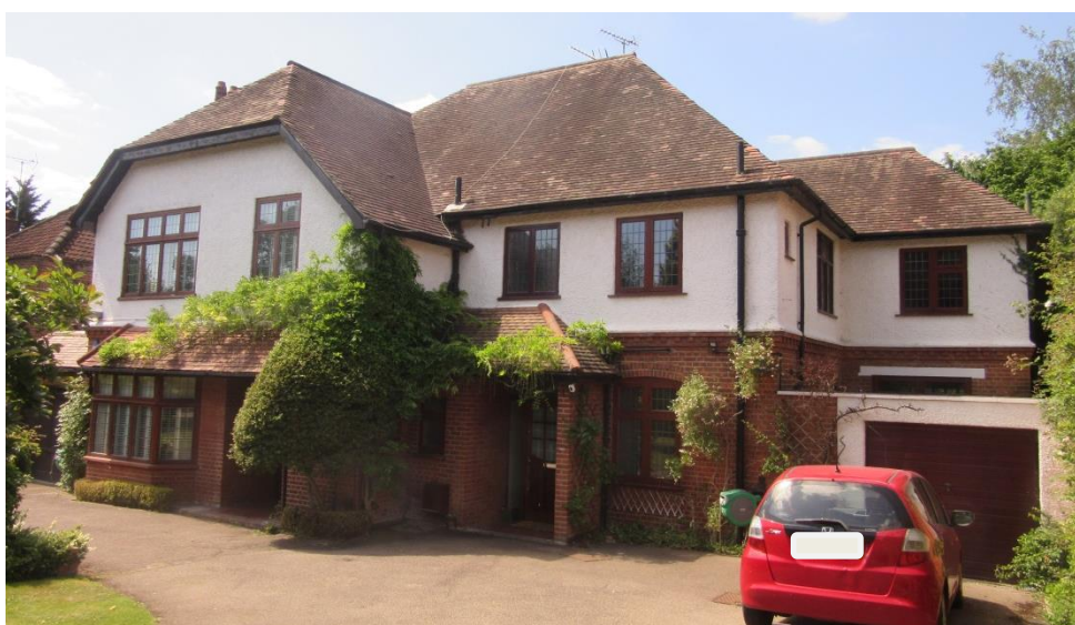
Figure 25: The front elevation of 11a View Road.
