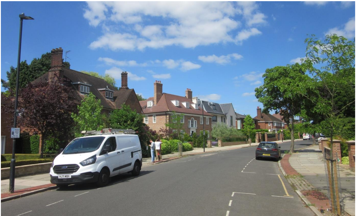
Figure 3: Sheldon Avenue looking north, including the replacement building at No. 23a (centre right).
