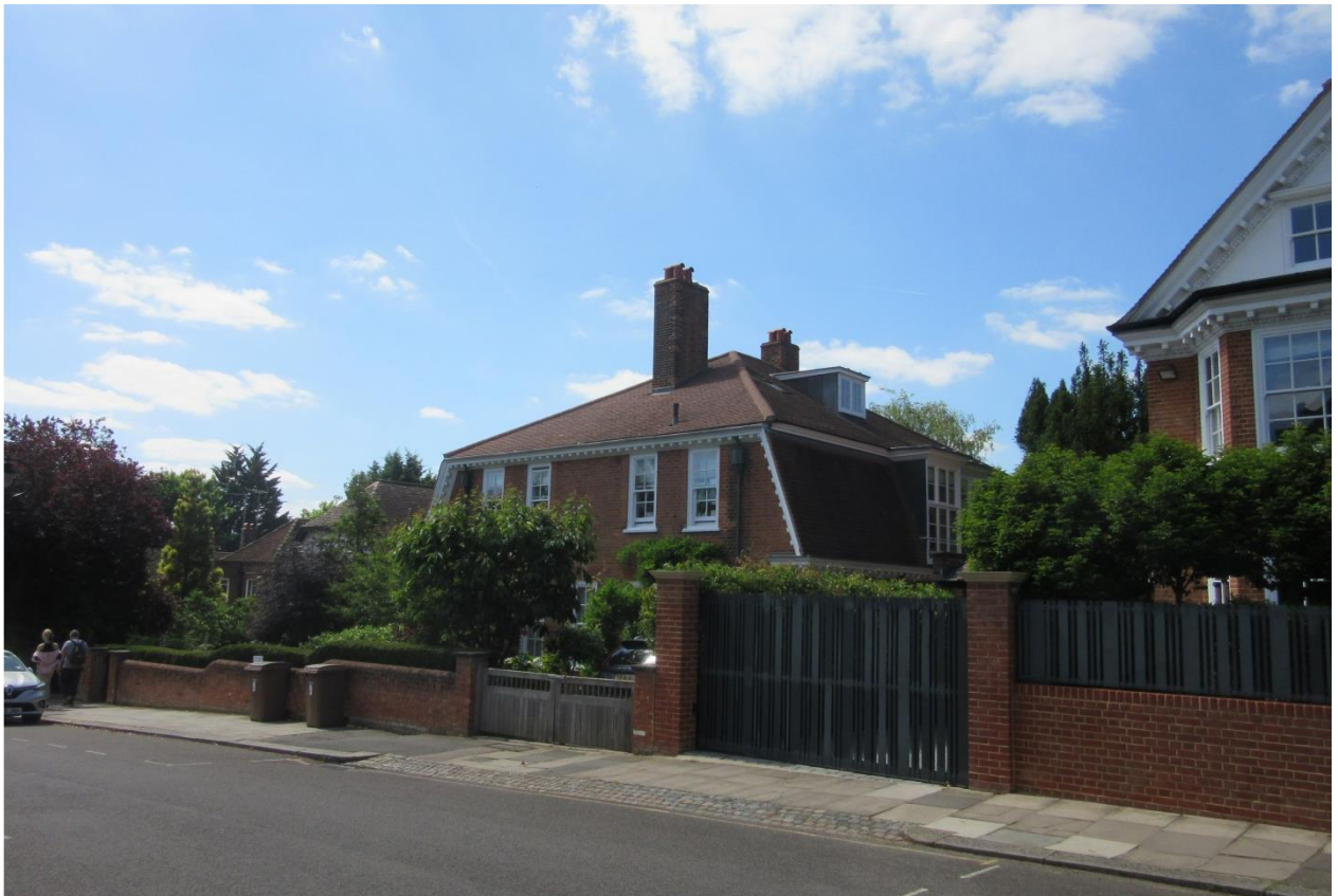
Figure 3a: View as existing from View Road looking south-west.
