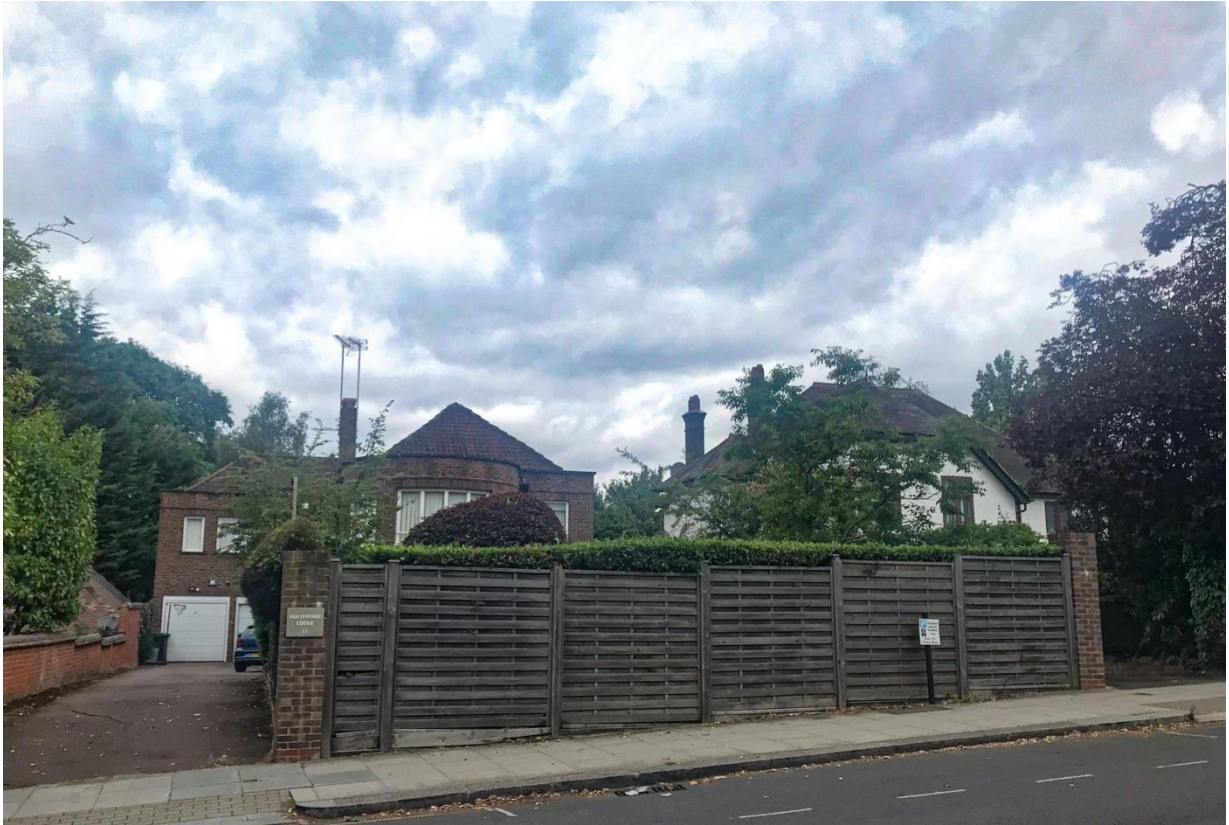
Figure 2a: View as existing north-east from View Road.
