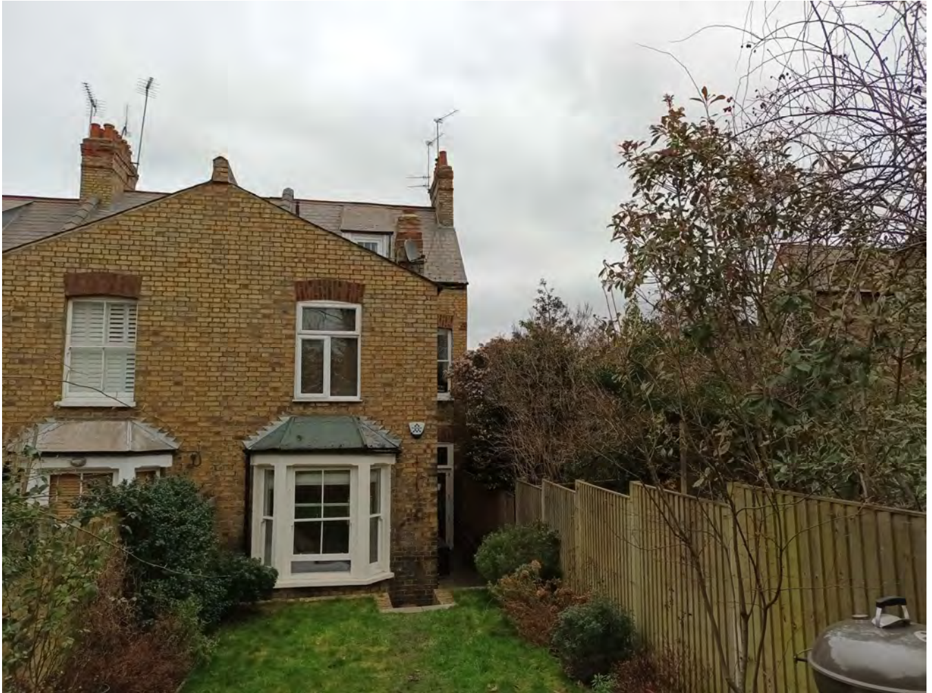
Photo 4 – Rear Elevation No1 Ferrestone Rd, indicating garden would be overlooked by roof terrace, plus boundary planting impacted by the proposals.
