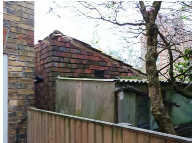
Photo 6 – Existing neighbour shed abutting garage
