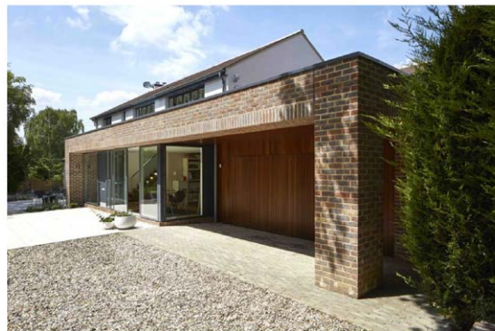
Brick frame entrance canopy
