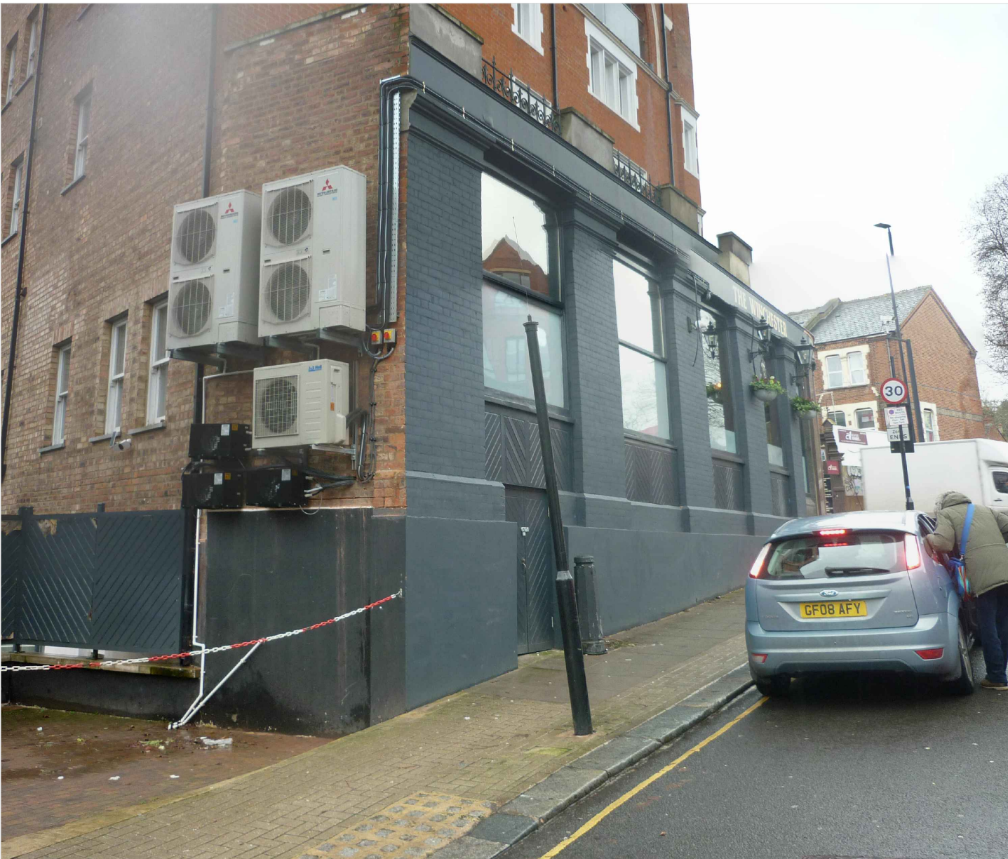
AC & Cellar cooling condensors as Existing
