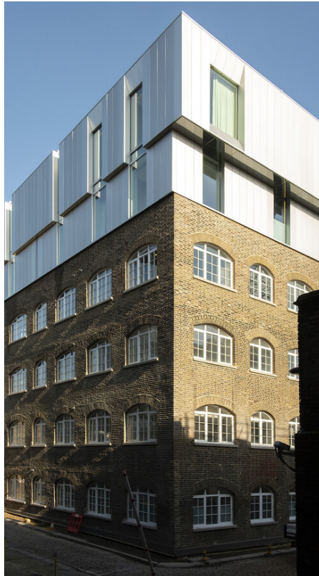
An example of stainless steel cladding to a roof extension in Camden. By Ambigram Architects.
