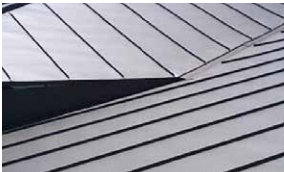
Metal cladding to shallow pitch roof
