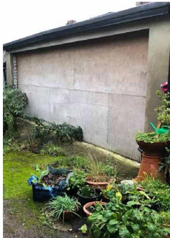
Rear elevation of existing garage to No. 97 Alexandra Park Road
