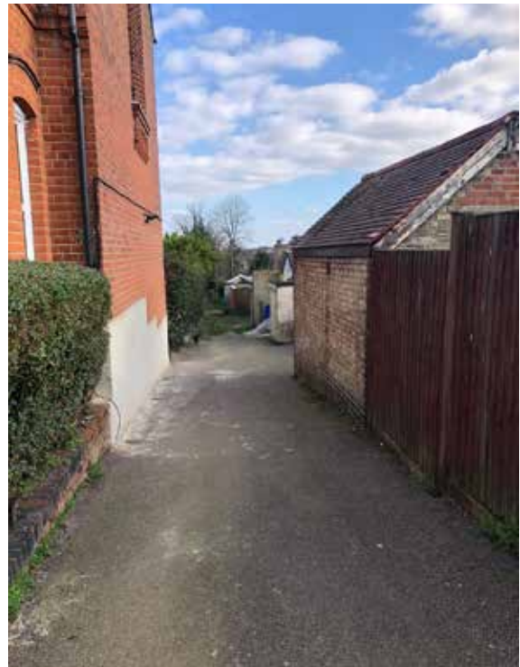
Outbuildings to rear of 85-107 Alexandra Park Road, accessed via Thirlmere Road
