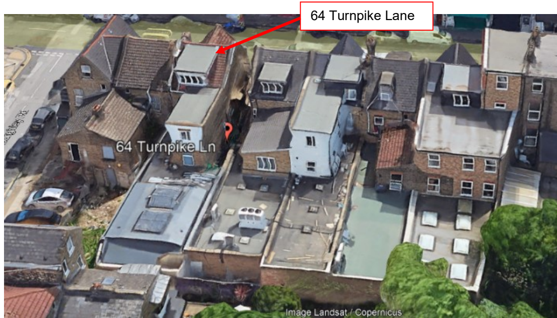
Aerial view of existing rear extensions 64- 72 Turnpike Lane
