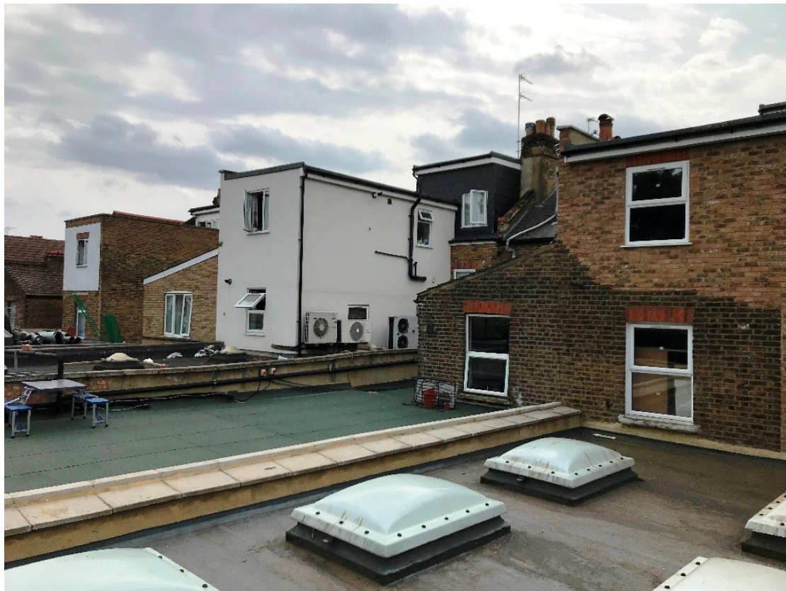
64-72 Turnpike Lane (Rear)
